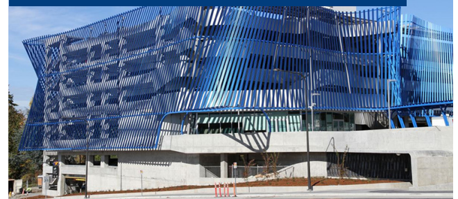
A building that is iconic and stands out (2.0 average rating)
