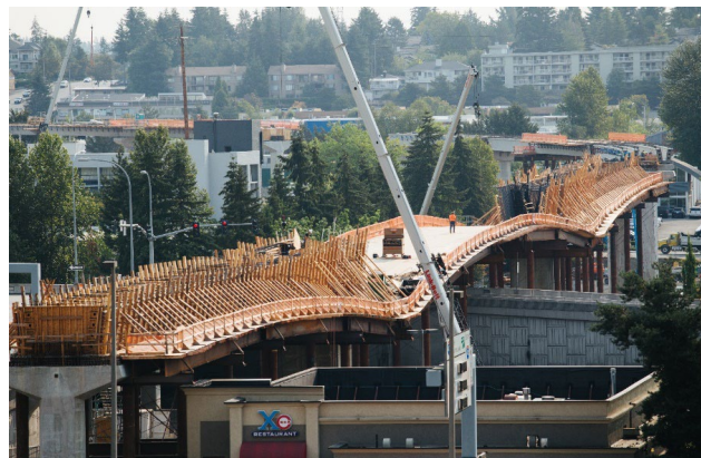
Figure 2-47. Construction of Elevated Guideway Over Roadways
