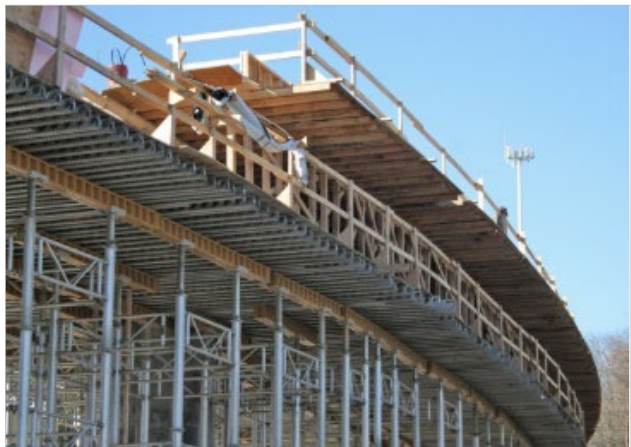
Figure 2-47. Construction of Elevated Guideway Over Roadways
