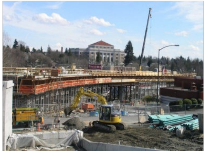
Figure 2-52. Staging Area Adjacent to New Guideway Under Construction
