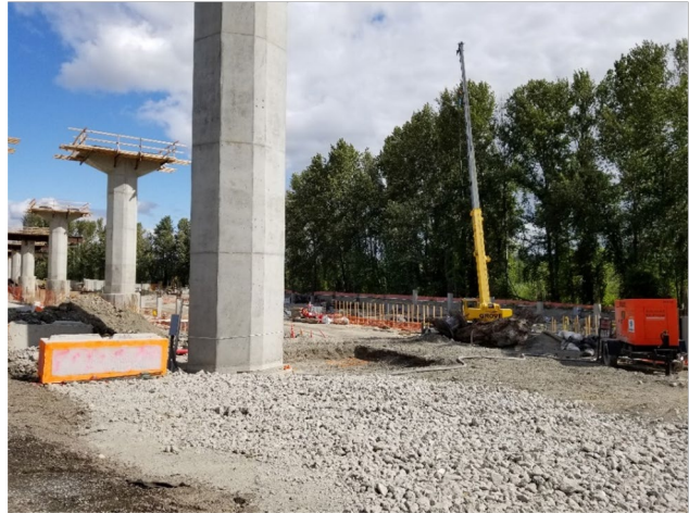
Figure 2-46. Construction of Elevated Guideway Showing False-work
