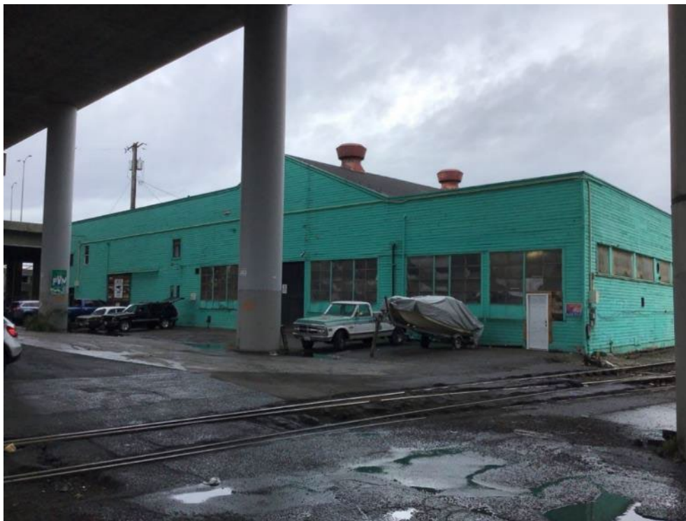
Figure N.5B-DUW-28. #1915, Alaskan Copper Works/Eagle Brass Foundry Company, 3600 East Marginal Way South (WISAARD #38532)
