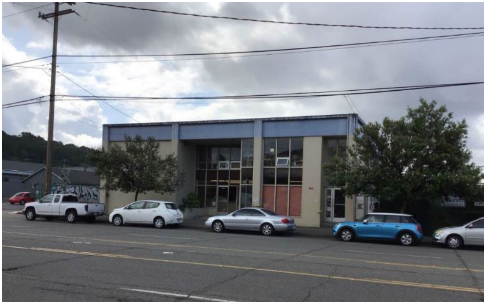
Figure N.5B-WSS-5. #2085a, Mill & Mine Supply Co. Building and Warehouse, 625 South Lander Street (WISAARD #343198)
