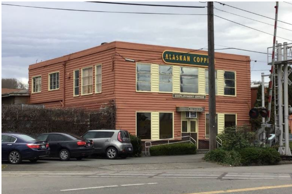
Figure N.5B-DUW-34. #3322a, Alaska Copper Co. Employment Office, 2958 6th Avenue South (WISAARD #342997)
