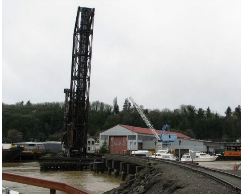
Figure N.5B-DUW-55. #LIN-12, Northern Pacific Railway Bridge Over the West Duwamish Waterway, South of Spokane Street, near Klickitat Way Southwest (WISAARD #44440)
