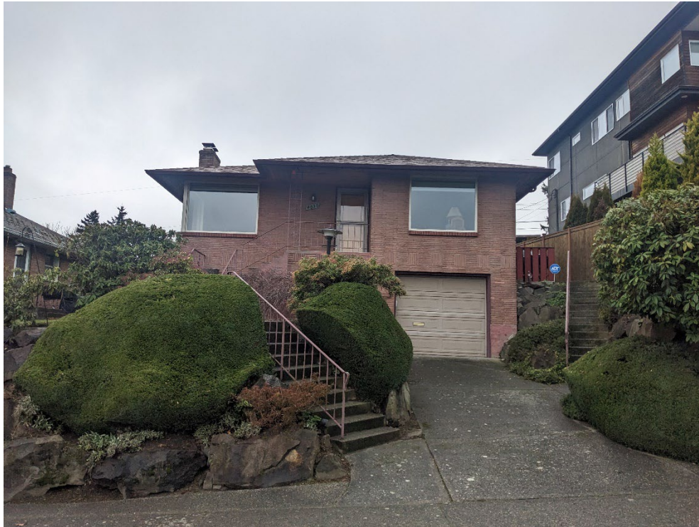
Figure N.5B-WSJ-28. #7010, Single-Family Residence, 4039 36th Avenue Southwest (WISAARD #729979)
