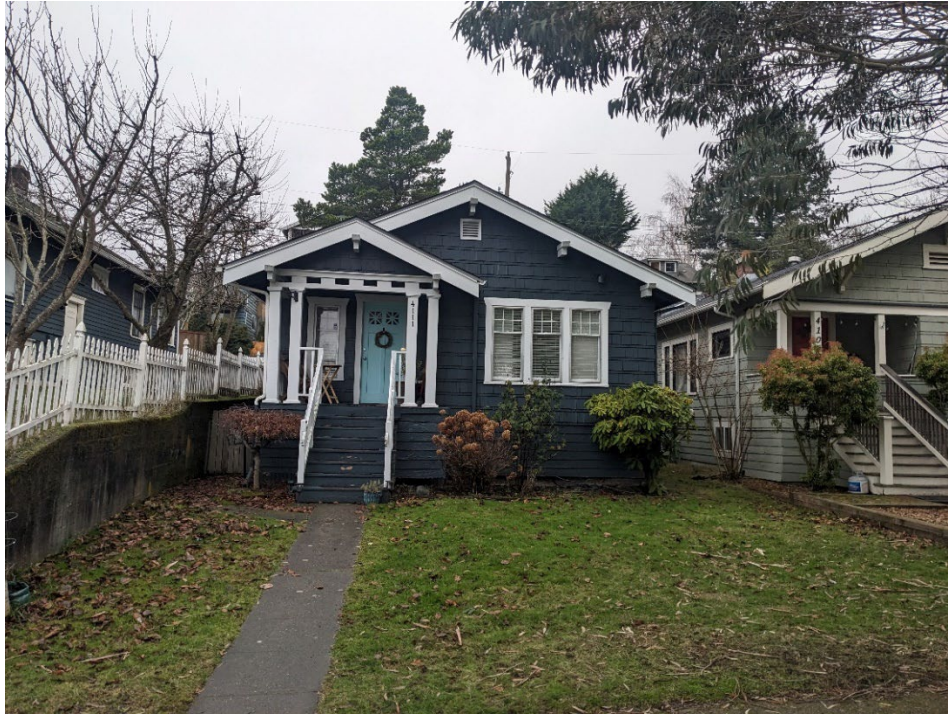
Figure N.5B-WSJ-31. #7053, Single-Family Residence, 4111 38th Avenue Southwest (WISAARD #730017)
