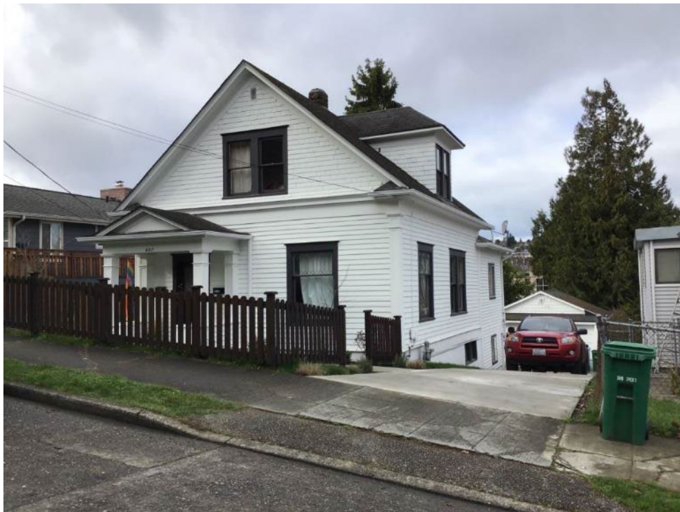
Figure N.5B-DEL-10. #3345, Residence, 4017 23rd Avenue Southwest (WISAARD #287692)
