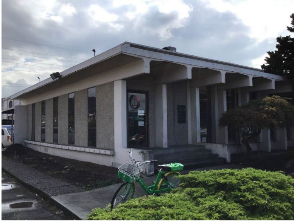
Figure N.5B-WSS-1. #1028, Lincoln Moving & Storage, Alaska Orient Van Lines Building, 1924 4th Avenue South (WISAARD #342325)
