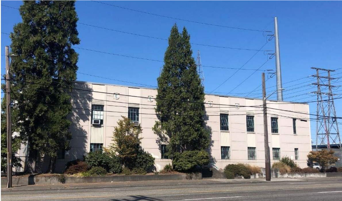
Figure N.5B-DUW-47. #5139a, Seattle City Light South Receiving Substation, 3839 4th Avenue South (WISAARD #45089)
