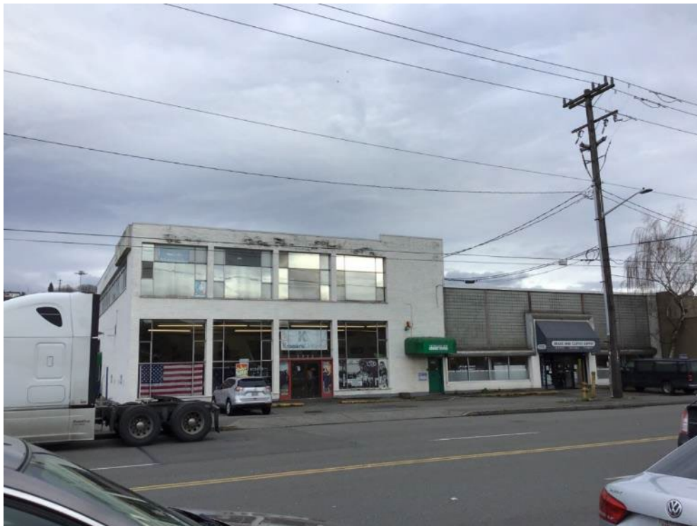
Figure N.5B-DUW-32. #3320b, NW Motor Parts Corporation Building, 2930 6th Avenue South (WISAARD #722007)
