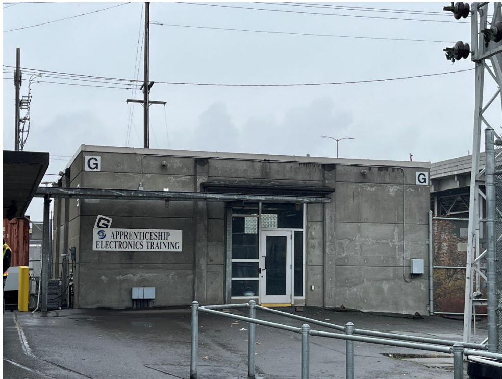
Figure N.5B-DUW-50. #5139e, Seattle City South Rectifier Substation, 3613 4th Avenue South (WISAARD #730784)
