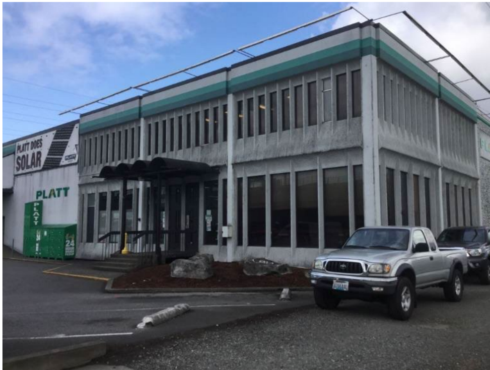
Figure N.5B-WSS-3. #1276, Platt Electric Supply Co., 2757 6th Avenue South (WISAARD #720594)
