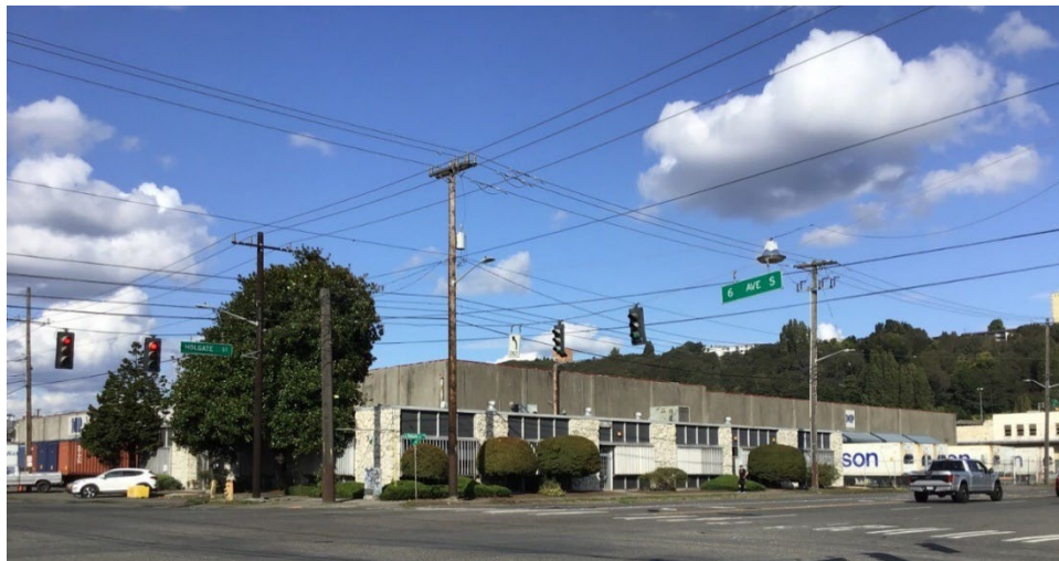
Figure N.5B-WSS-4. #1899, Holgate Terminals Incorporated, 1762 6th Avenue South (WISAARD #342236)
