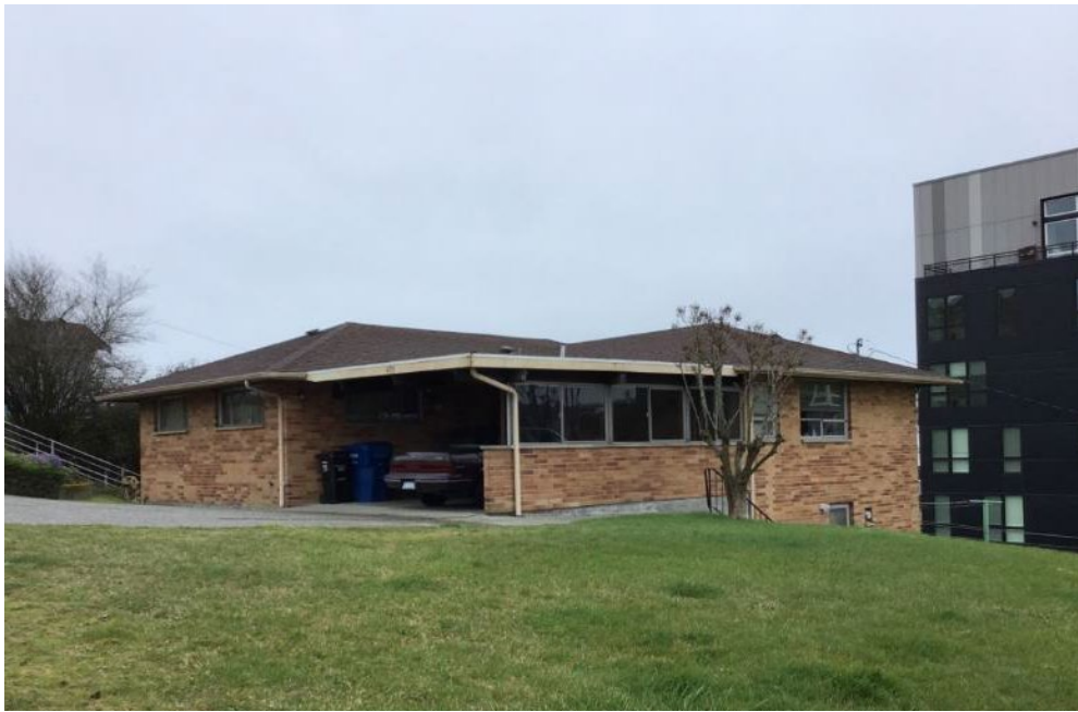
Figure N.5B-WSJ-25. #3250, Single-Family Residence, 4755 38th Avenue Southwest (WISAARD #722762)
