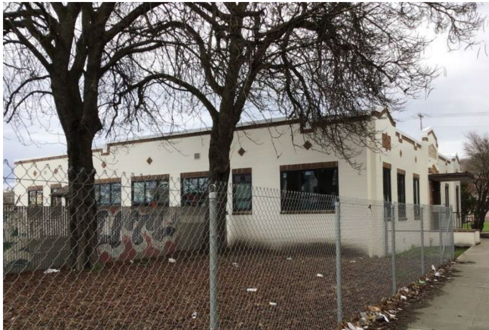
Figure N.5B-DUW-38. #3329a, Department of Highways District No. 1 Headquarters/Maintenance Facility - Office/Administrative Building, 450 South Spokane Street (WISAARD #86871)
