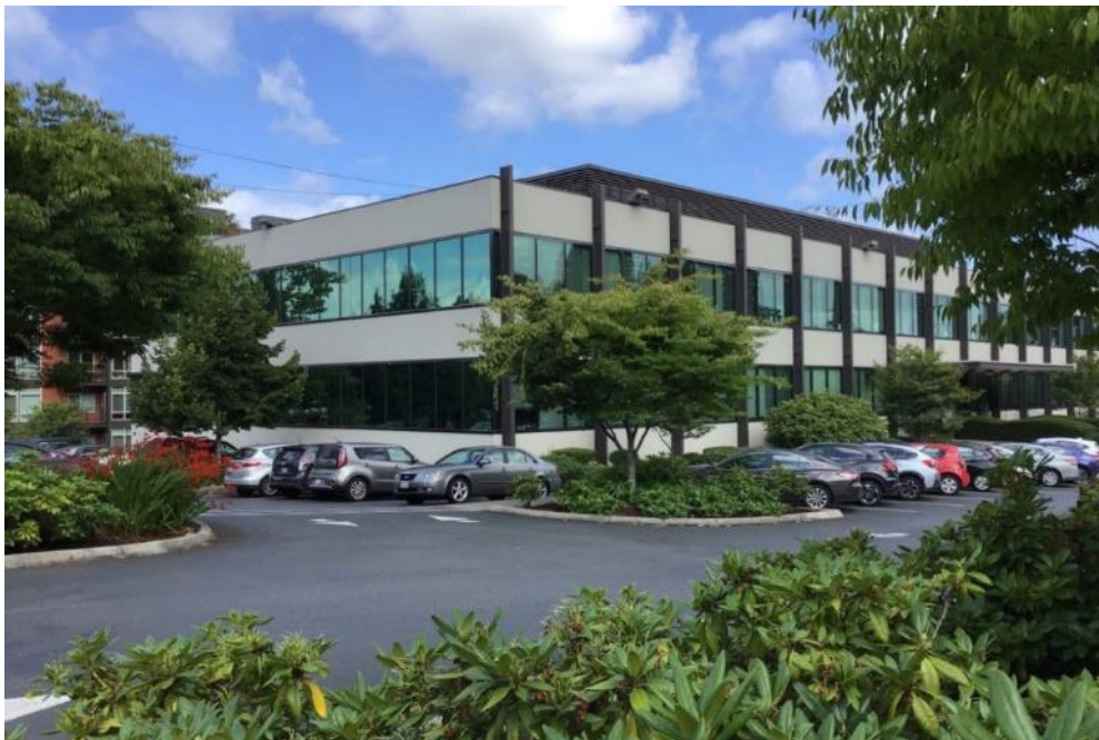
Figure N.5B-DEL-2. #443, Bethlehem Pacific Coast Steel Company Office Building, 4045 Delridge Way Southwest (WISAARD # 344641)
