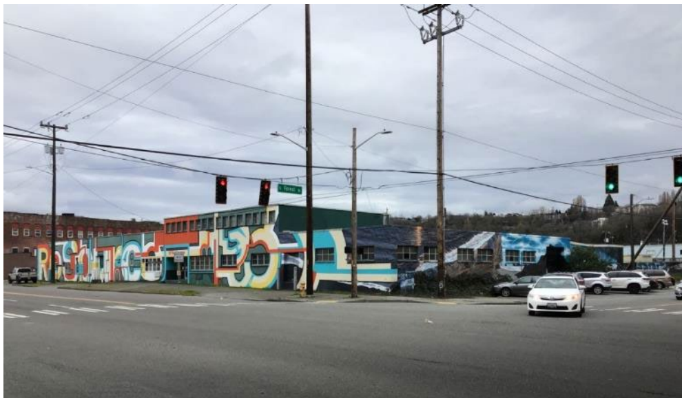
Figure N.5B-WSS-6. #3317, Northwest Wire Works, 2752 6th Avenue South (WISAARD #721855)
