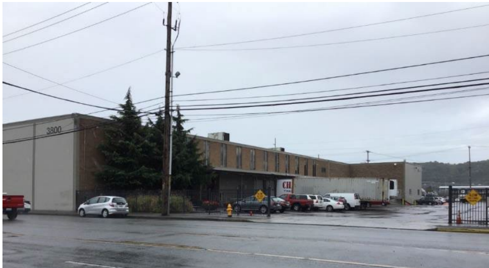
Figure N.5B-DUW-2. #881, Seattle Pacific Sales Company Warehouse, 3800 1st Avenue South (WISAARD # 342274)
