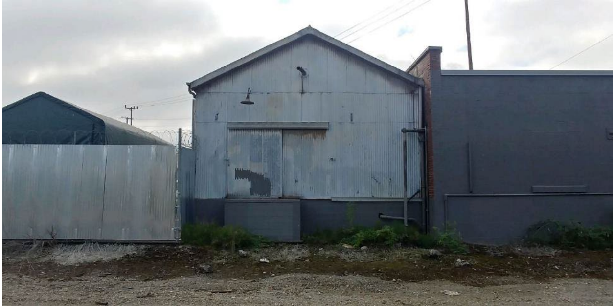
Figure N.5B-DUW-13. #1103b, Air Reduction Company Carbide Storage Building, 3621 East Marginal Way South (WISAARD # 720563)
