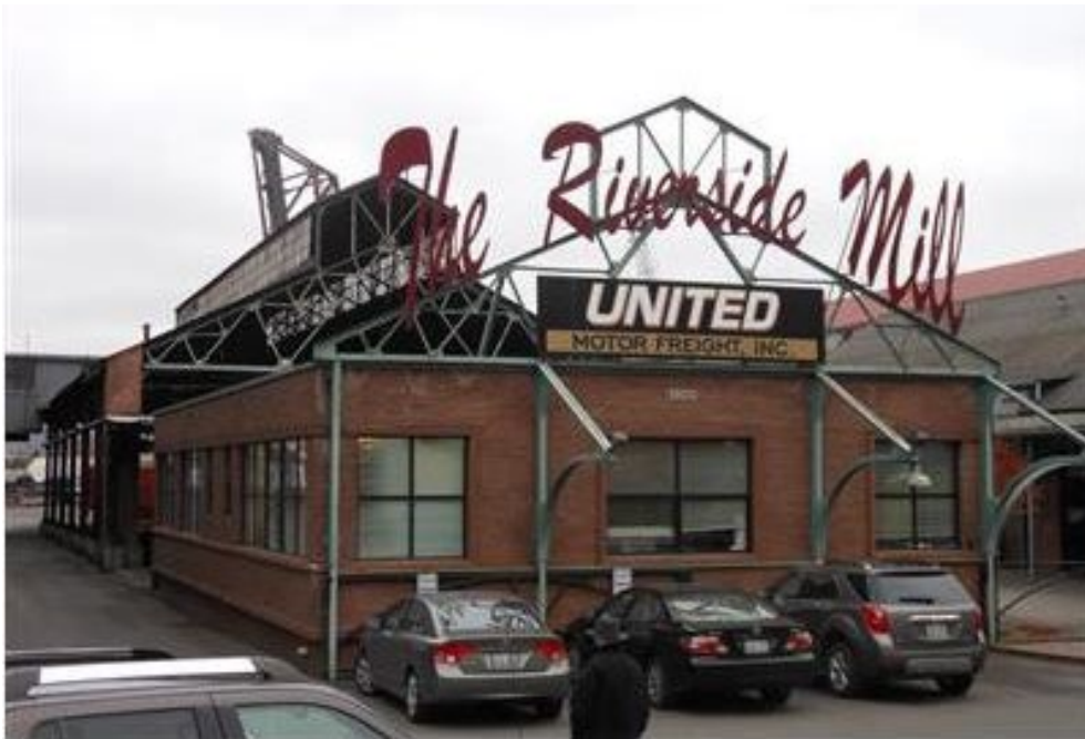
Figure N.5B-DUW-17. #1122a, Pacific Forge Company/Bethlehem Steel Nut and Bolt Factory Office, 3800 West Marginal Way Southwest (WISAARD #721620)
