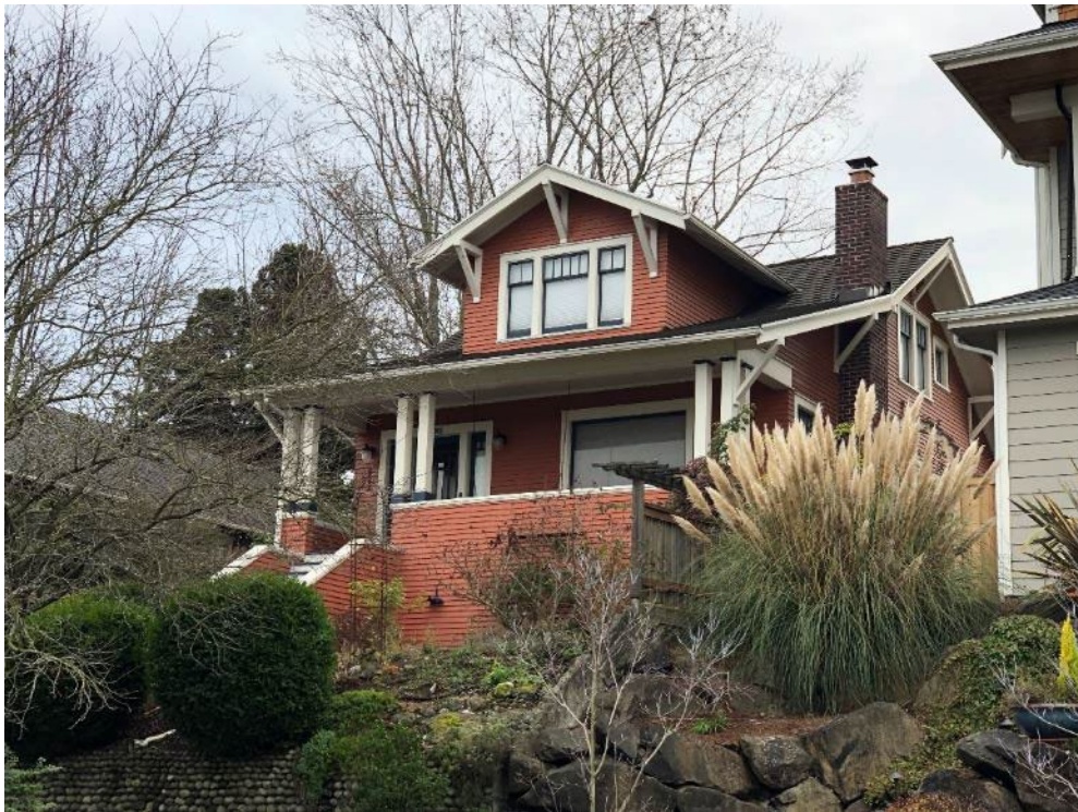
Figure N.5B-WSJ-19. #2224, Residence, 5011 41st Avenue Southwest (WISAARD #721512)
