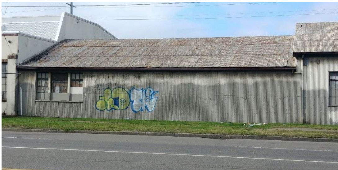
Figure N.5B-DUW-40. #3329c, Department of Highways District No. 1 Headquarters/Maintenance Facility - Storage Building, 450 South Spokane Street (WISAARD #722098)
