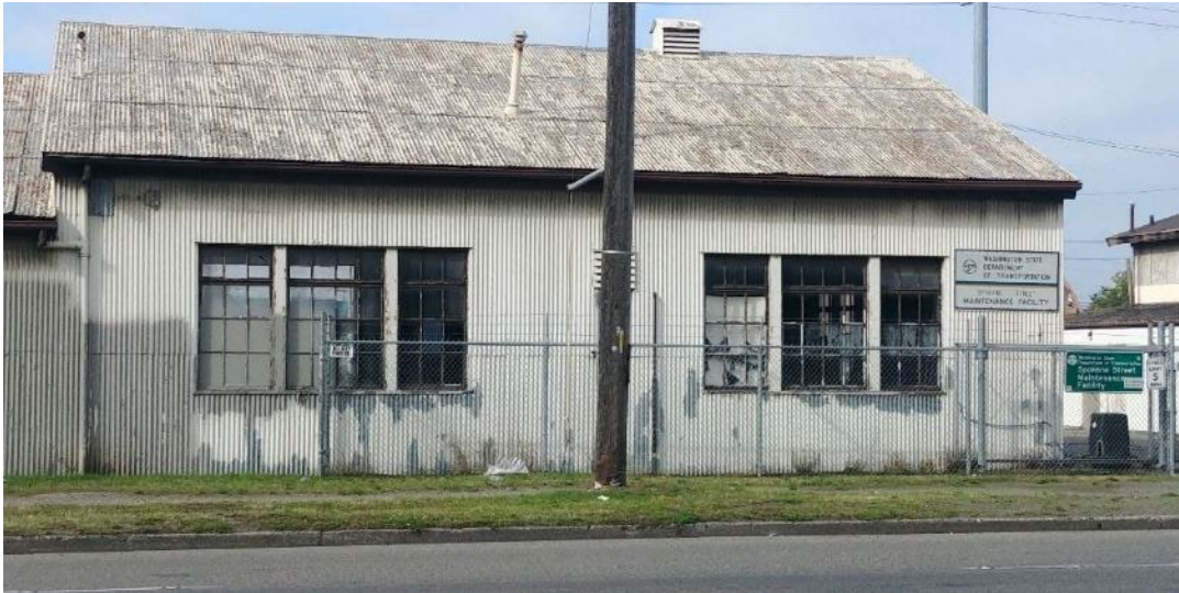
Figure N.5B-DUW-41. #3329d, Department of Highways District No. 1 Headquarters/Maintenance Facility - Car/Paint Building, 450 South Spokane Street (WISAARD #722100)
