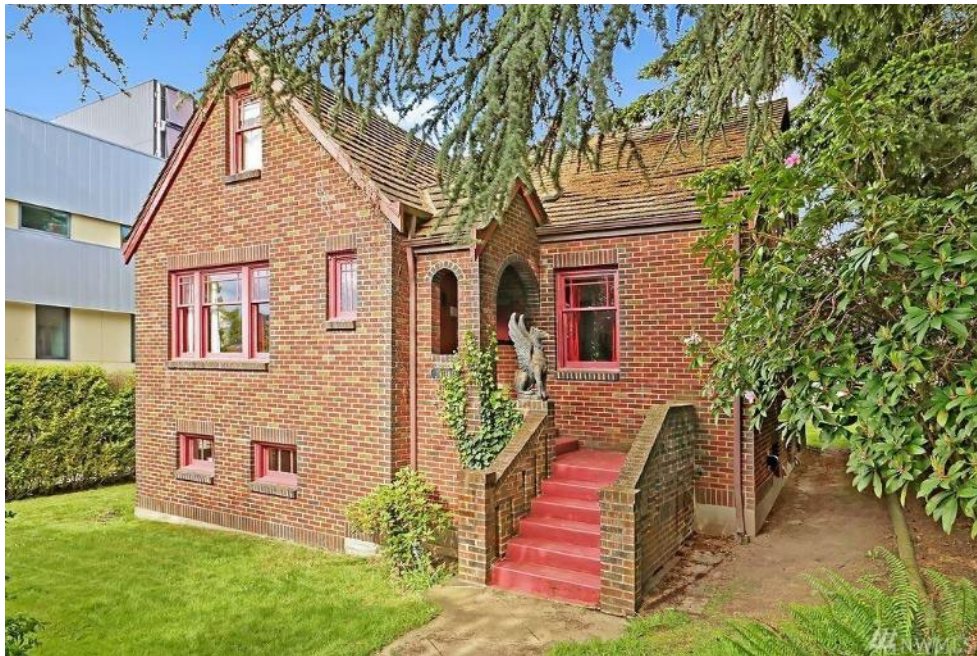
Figure N.5B-WSJ-24. #3243, Single-Family Residence, 4714 38th Avenue Southwest (WISAARD #722760)
