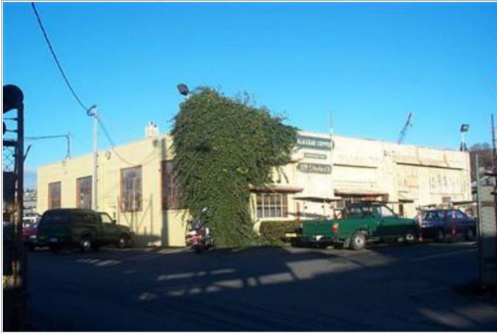
Figure N.5B-DUW-35. #3322b, Auto Repair Garage, 2958 6th Avenue South (WISAARD #721997)
