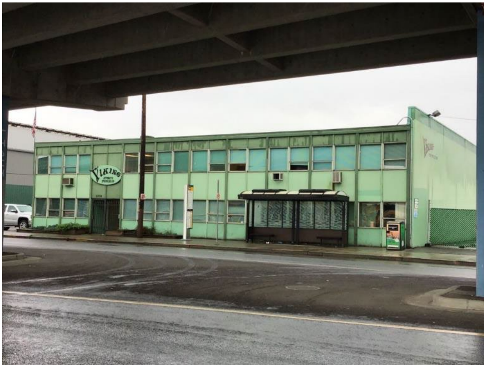
Figure N.5B-DUW-4. #1083, Viking Automatic Sprinkler Company, 3434 1st Avenue South (WISAARD #718431)
