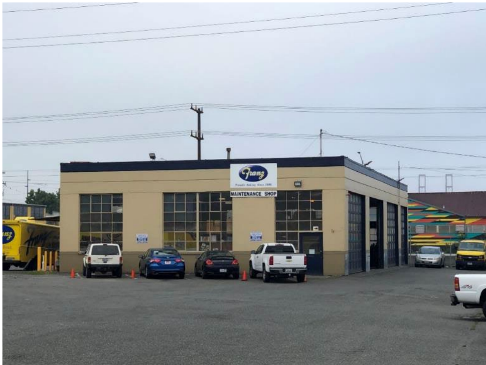
Figure N.5B-DUW-26. #1275b, Langendorf United Bakeries Repair Garage, 2901 6th Avenue South (WISAARD #720593)
