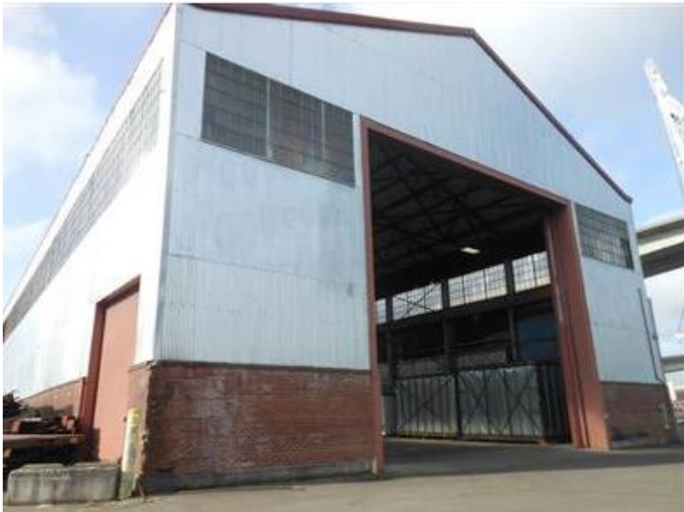
Figure N.5B-DUW-20. #1122d, Pacific Forge Company/Bethlehem Steel Nut and Bolt Factory South Warehouse, 3800 West Marginal Way Southwest (WISAARD #721628)
