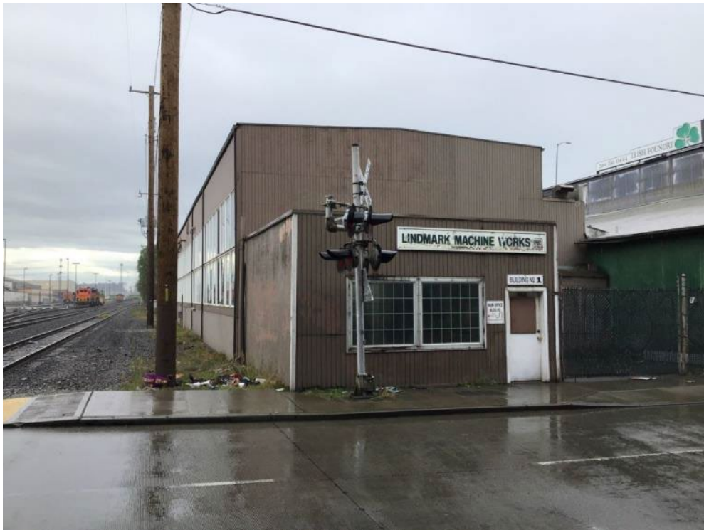
Figure N.5B-DUW-11. #1095, Lindmark Machine Works, 49 South Spokane Street (WISAARD # 340118)
