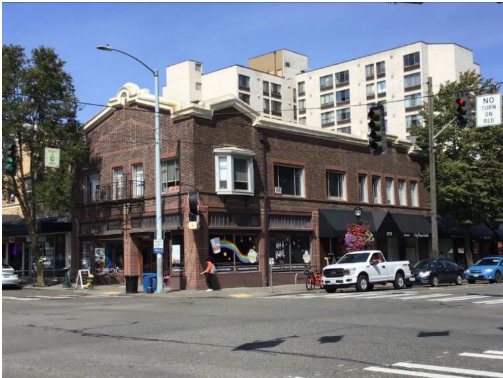
Figure N.5B-WSJ-6. #177, Campbell Building, 4554 California Avenue Southwest (WISAARD #721552)
