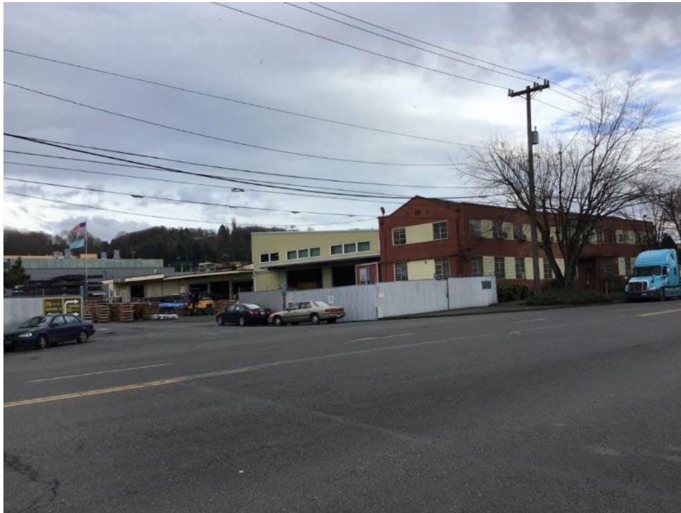
Figure N.5B-DUW-36. #3324, Los Angeles-Seattle Motor Express Company, 3200 6th Avenue South (WISAARD #340010)
