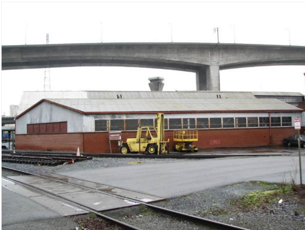
Figure N.5B-DUW-18. #1122b, Pacific Forge Company/Bethlehem Steel Nut and Bolt Factory Pacific Coast Forge Building (Original Forge buildings), 3800 West Marginal Way Southwest (WISAARD #721624)
