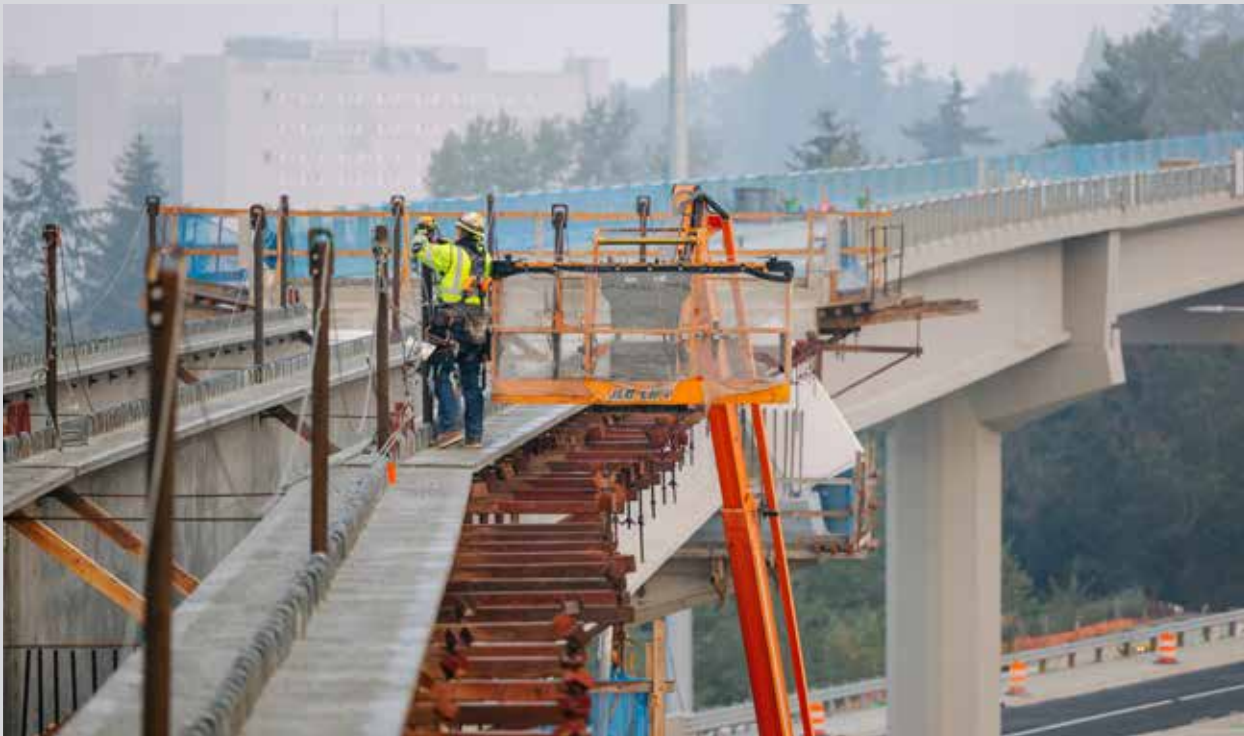
Federal Way construction
