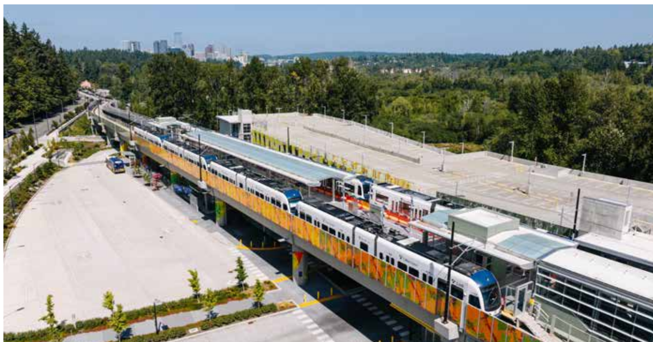
Testing trains for the new 2 Line. Sound wall mural by Vicki Scuri Siteworks with Alex Pozlin (fabricated by Winsor Fireform, Tumwater, Washington)
