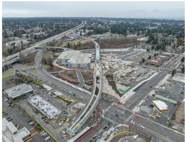
An aerial view of Lynnwood City Center Station and its adjacent bus loop and parking garage.
