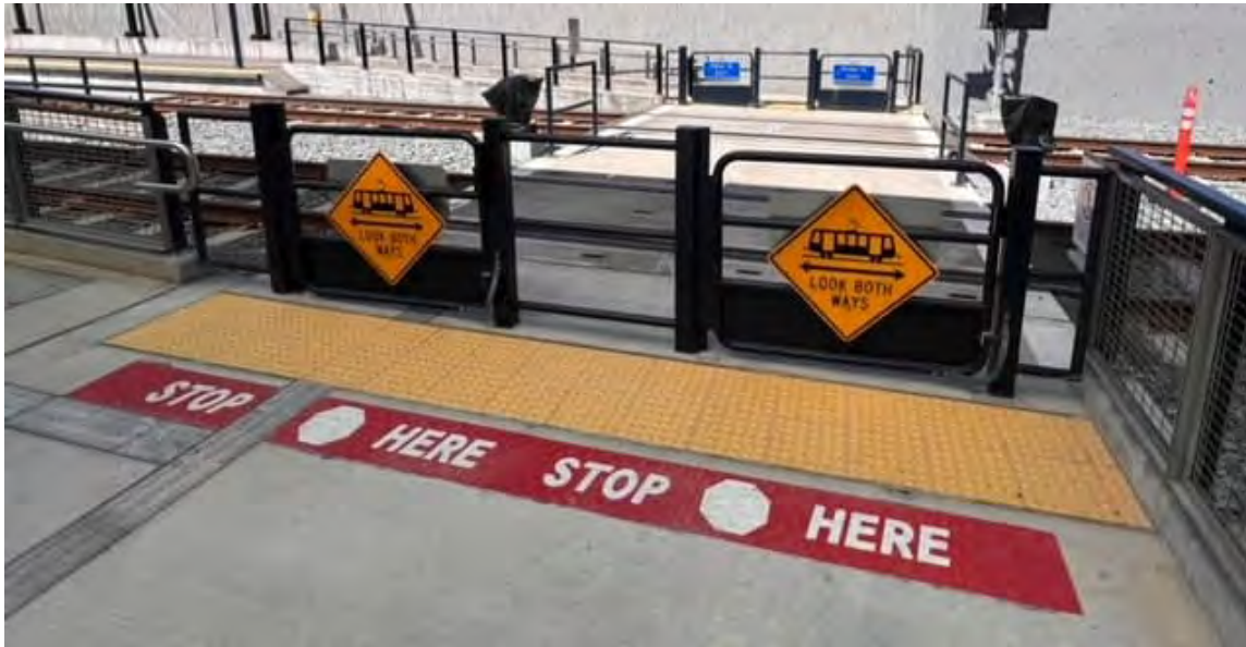
Figure 120-22: Pedestrian Swing Gate (rear view from track side)
