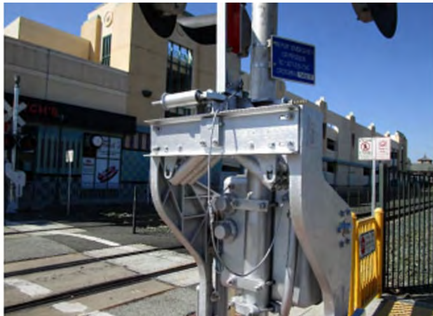
Figure 120-5: Gate Keeper Assembly
