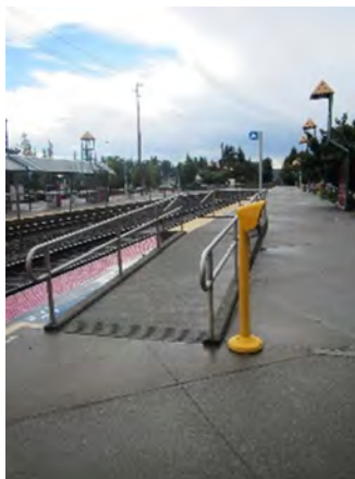
Figure 821-3: Typical Sounder Mini-high Platform, Sumner Station
