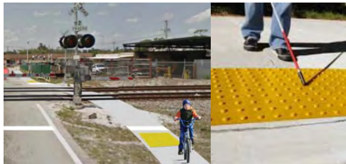
Figure 120-27: Detectable Warning Surface
