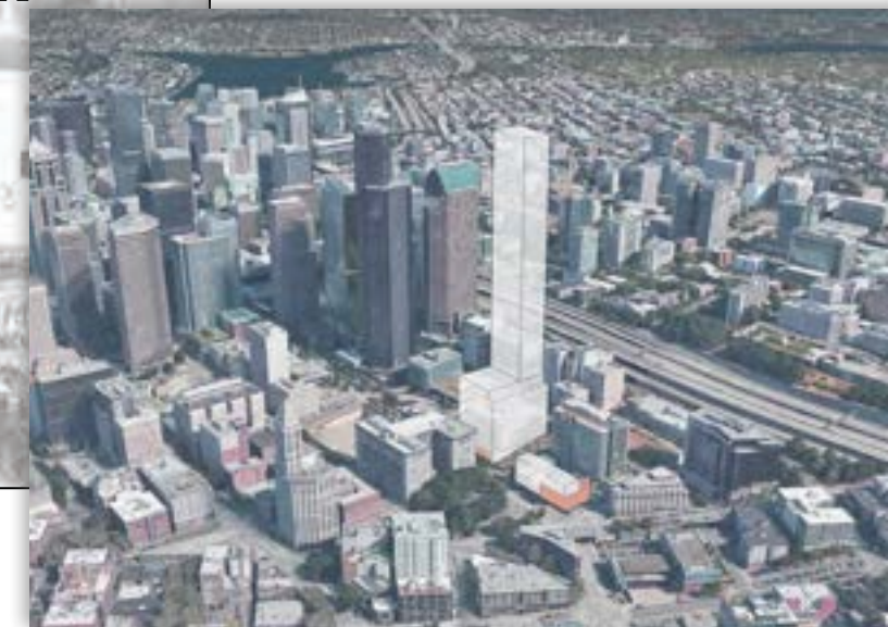
View to north of transit-oriented development sites with up to 1,700 homes and 400,000 square feet of commercial space
