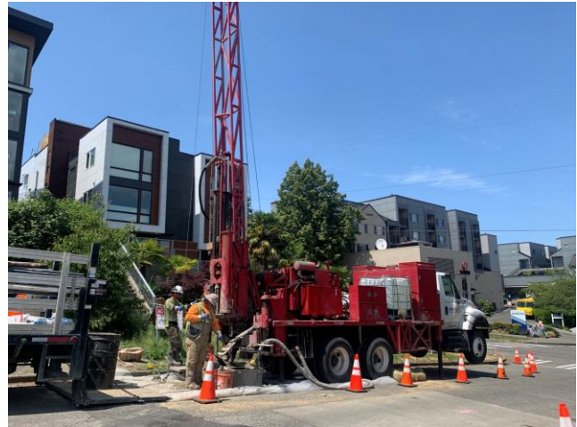
Example of geotechnical drilling equipment
