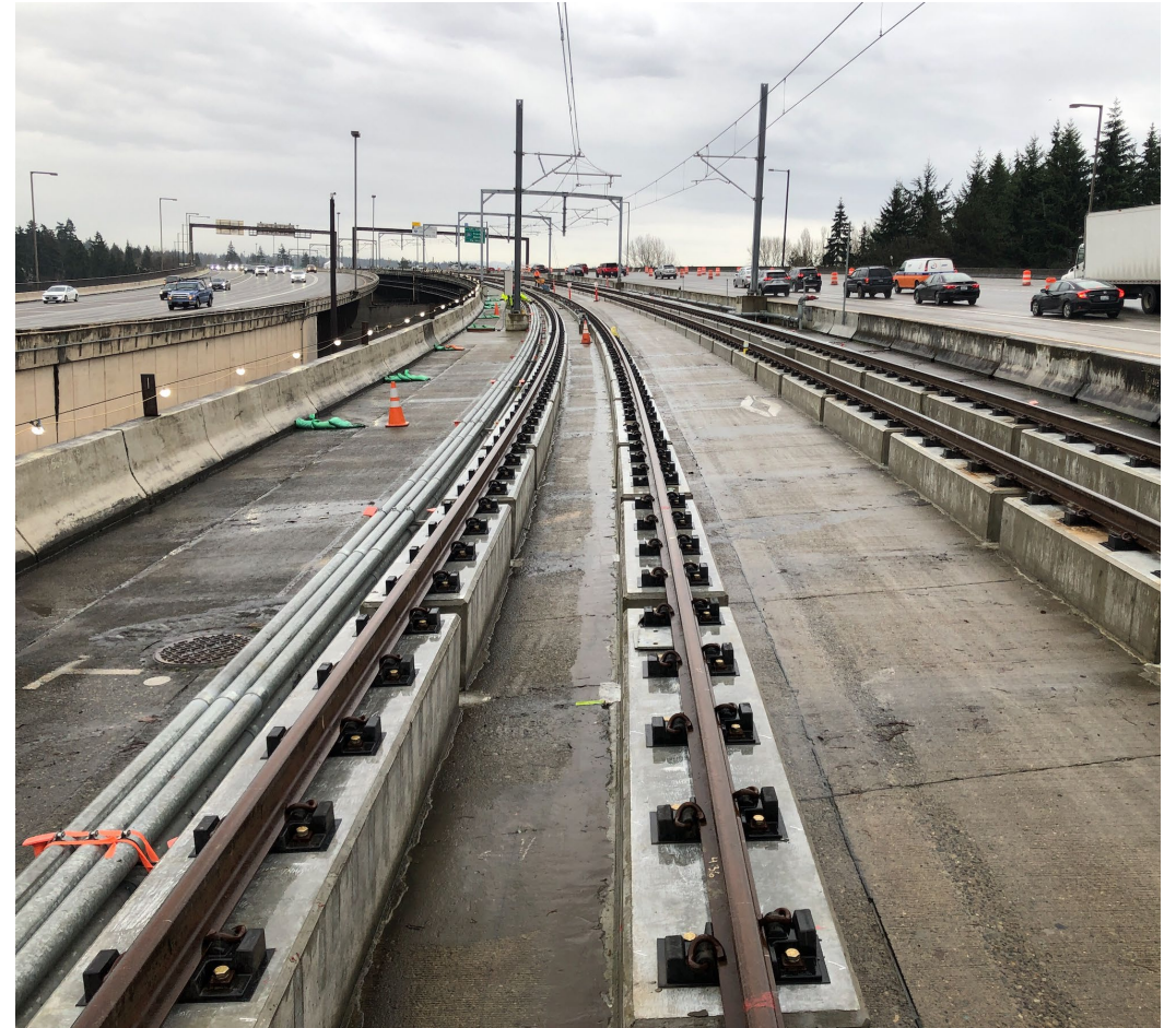
Completed Track on East Channel Bridge Looking West
