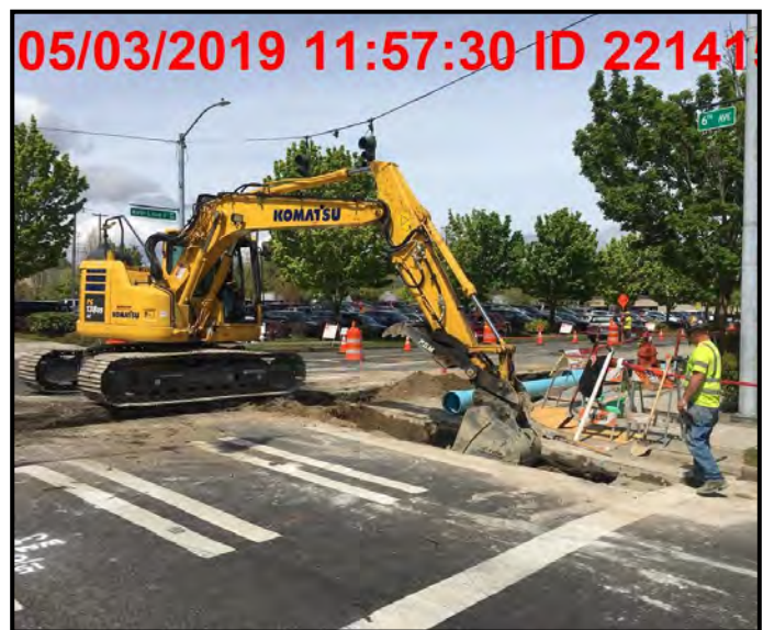
Water crew continues trenching work.
