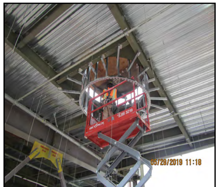
RVS— Installation of Skylights at North Entrance.
