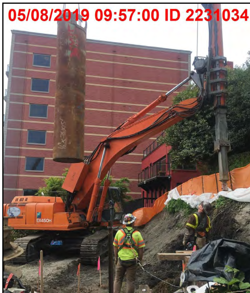
Inserting casing into shaft for Pile 9.
