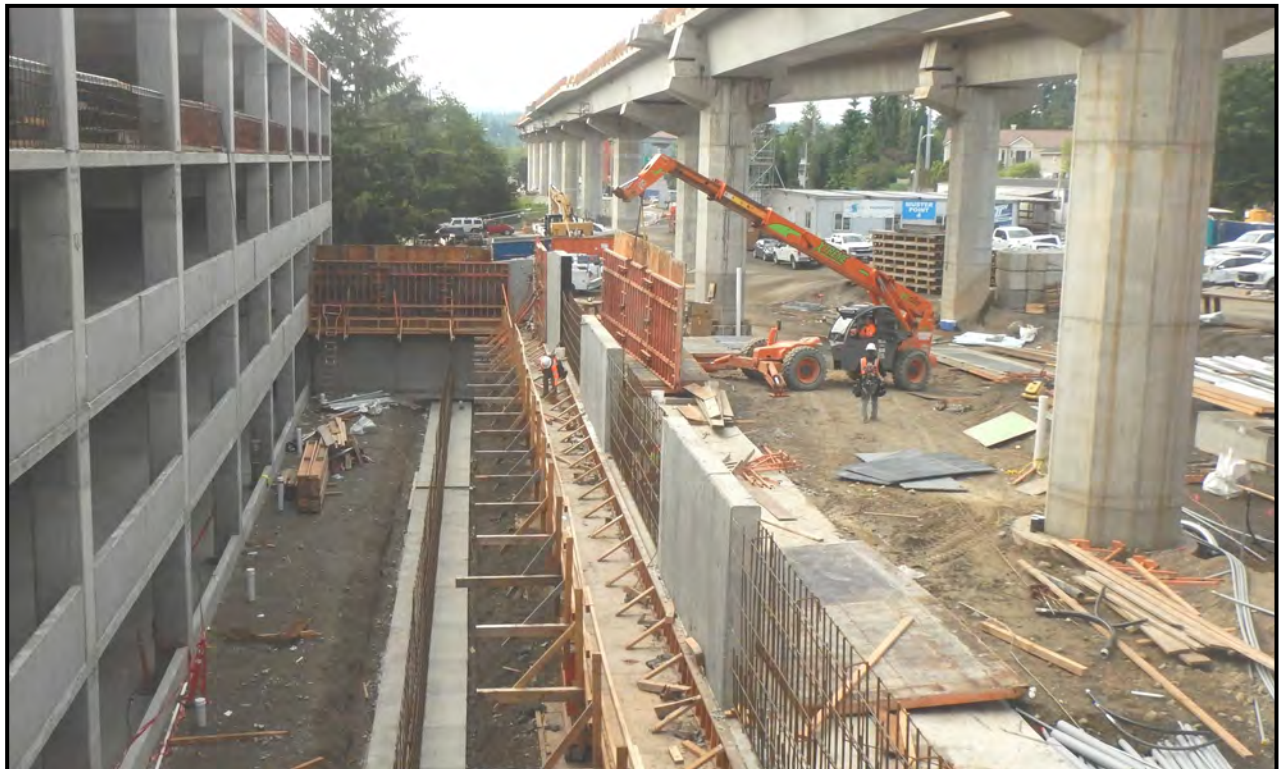
E320 South Bellevue: Setting wall forms for concrete pour.
