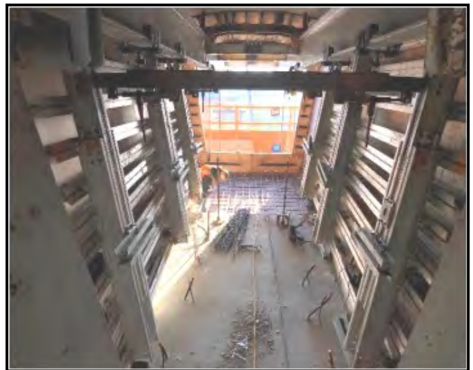
Topside look from within the Traveler system working over I-90
