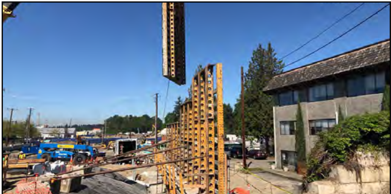
E340 Bel-Red : Installing wall panel facing west.
