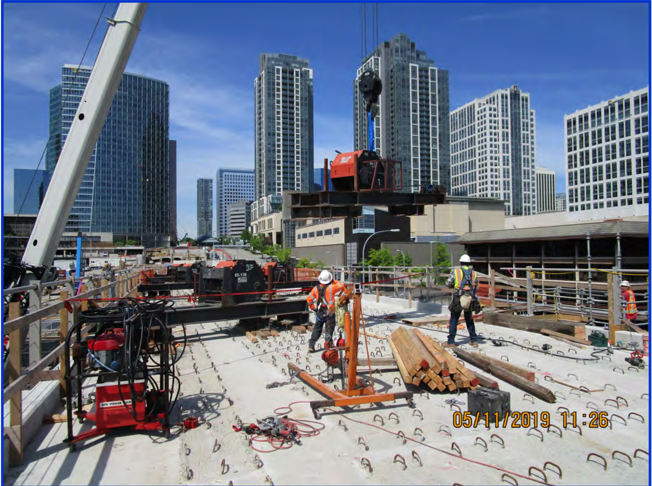
Long Span Falsework Removal (East Link)
