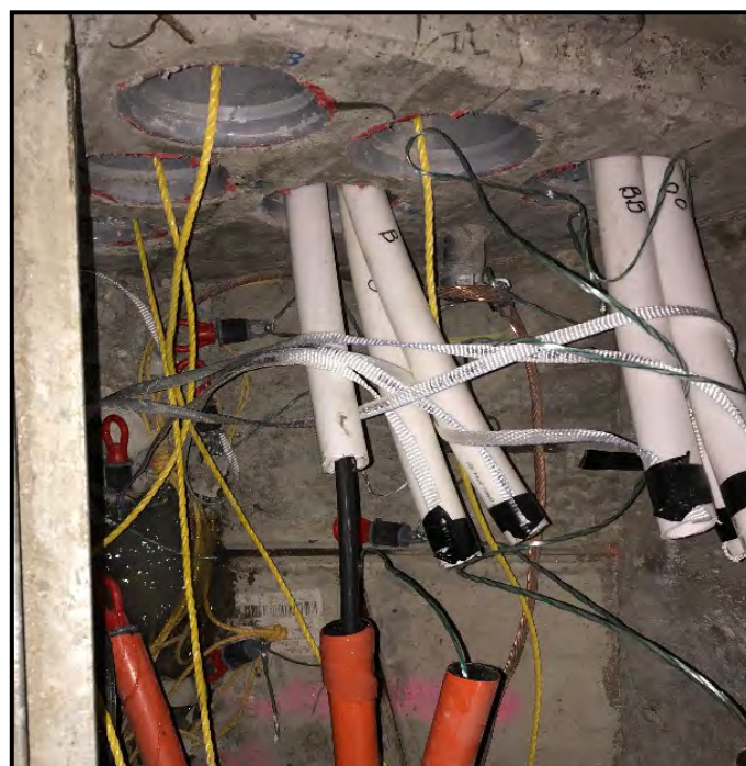
Pulling Fiber Cable from UDS to RVS, May 2, 2019
