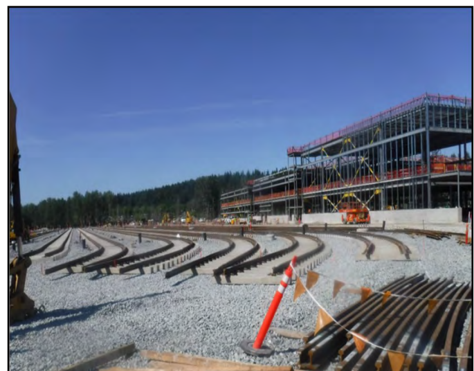
Curved Rail Installation and Exterior Wall Framing OMFE
