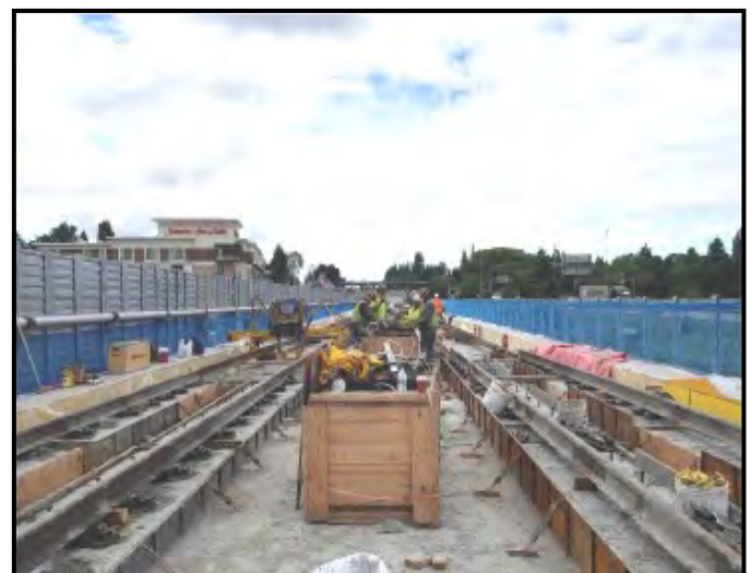
SWI - A view (facing south) of the completed plinths.
