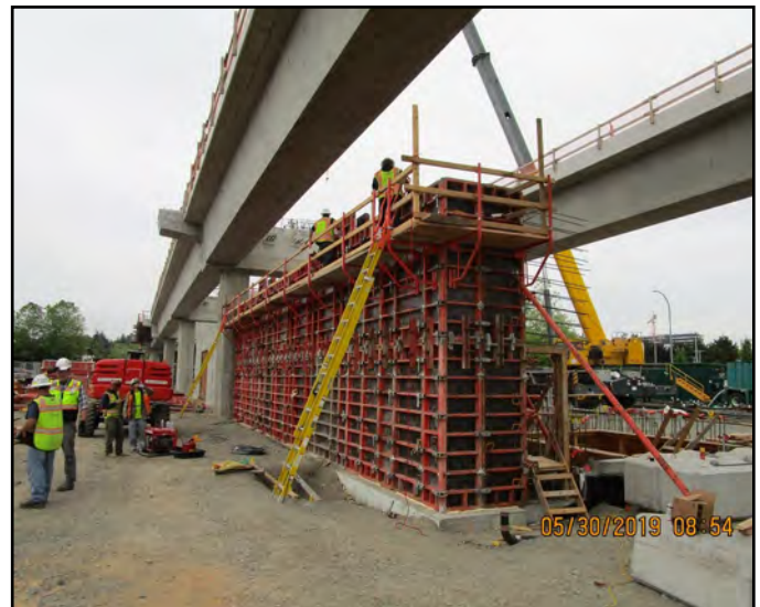
Wall forms at Wilburton Station. (Area 4)
