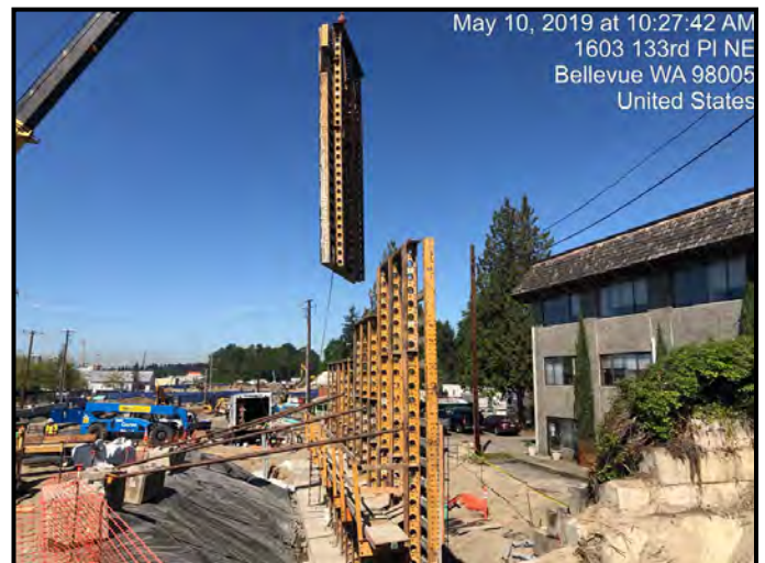
Installing a wall panel facing west at the station area.
