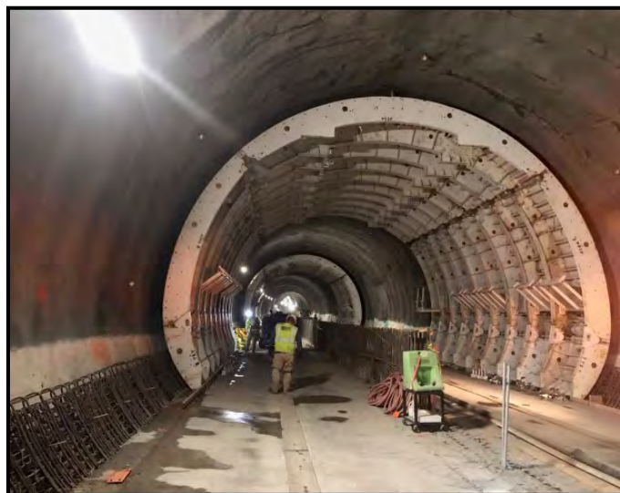
Final lining tunnel forms staged in the Tunnel.
