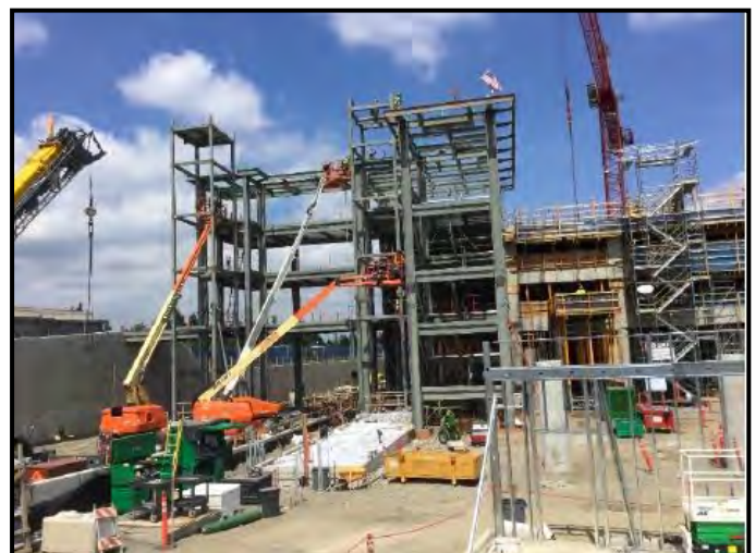
Work Area 6 - Vertical Circulation Tower at Redmond Technology Station
