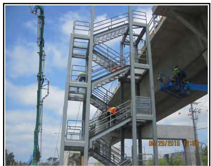
American Ironworkers crew installing railing at Station Maintenance Stair.
