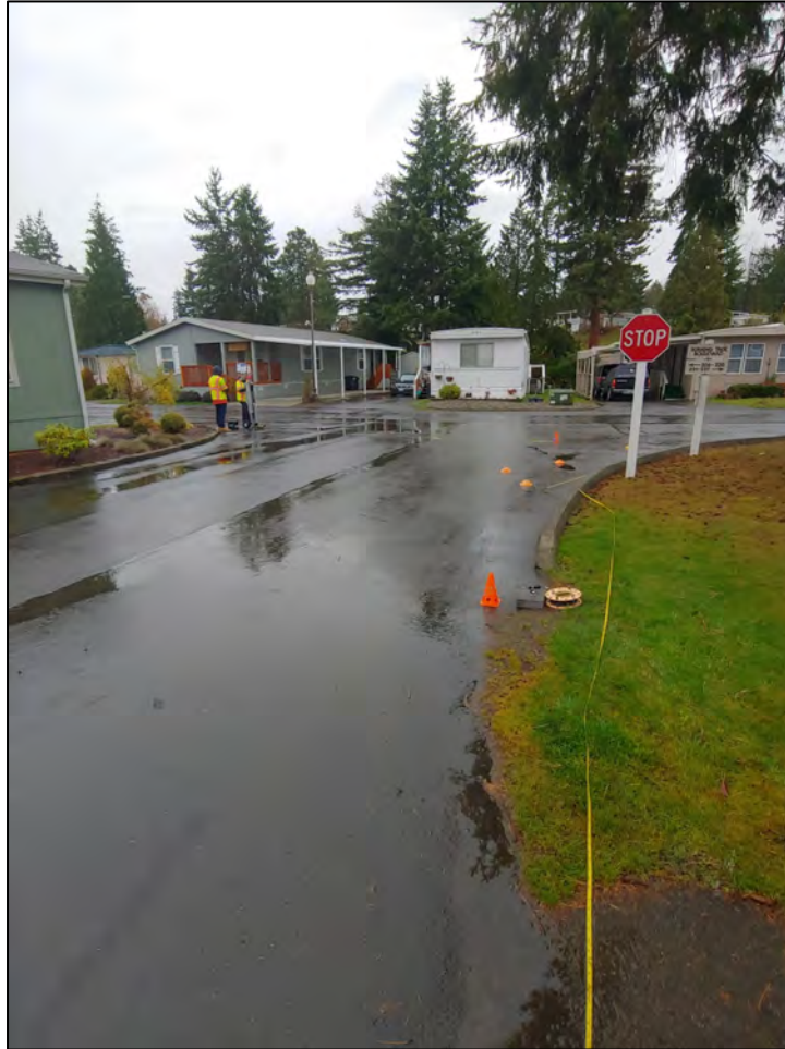
Figure G2-1.9 Vibration Propagation Measurement: Belmor Mobile Home Park
