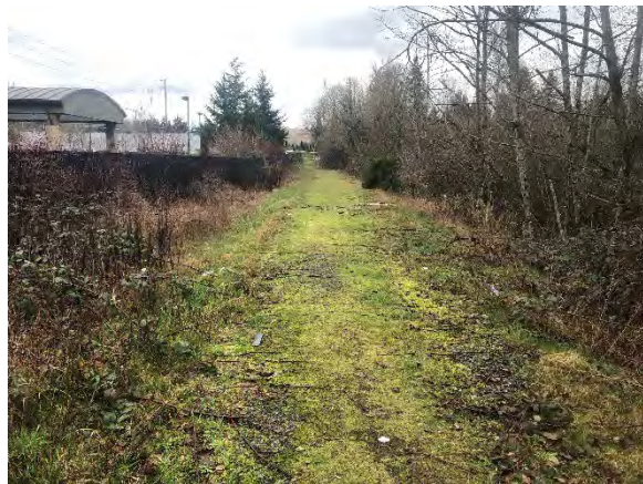
Figure G4.6-8 View of the levee along the western boundary of OMF 152, view north
