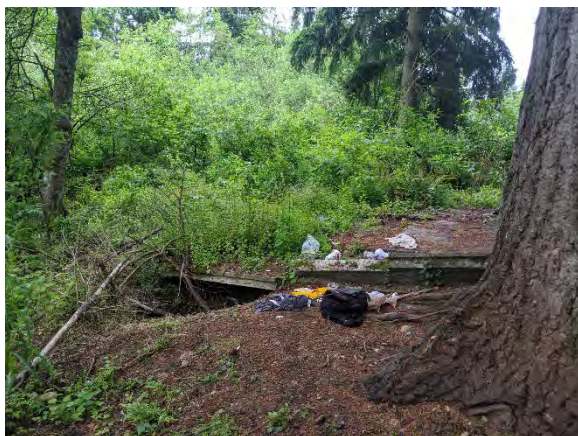
Figure G4.6-28 Concrete pad with disturbed perimeter foundation, view southeast
