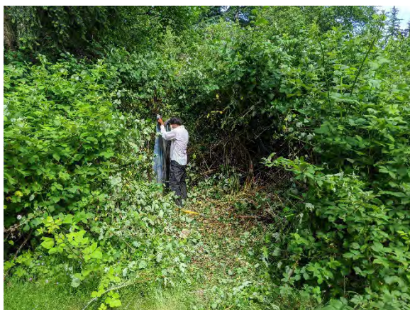
Figure G4.6-30 Cleared vegetation for excavation (SP01-17), view northeast
