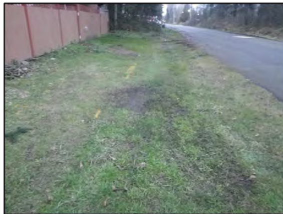
Figure G4.6-19 Marked buried natural gas pipeline (yellow paint) on the west side of 24th Avenue S, view north
