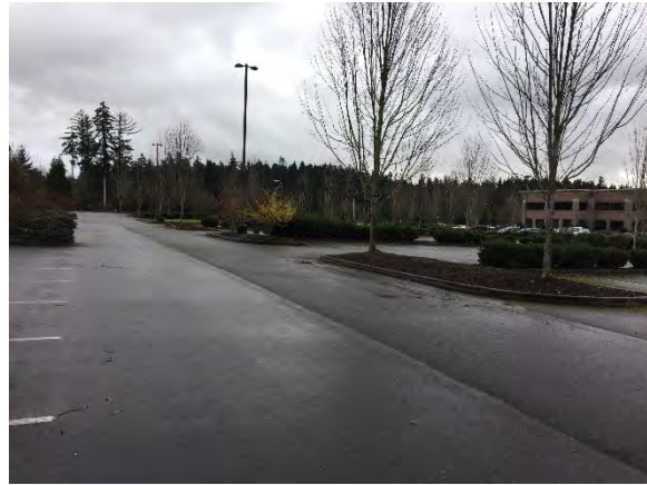
Figure G4.6-6 Paved areas partially surrounded by ornamental green space, OMF 151, view west
