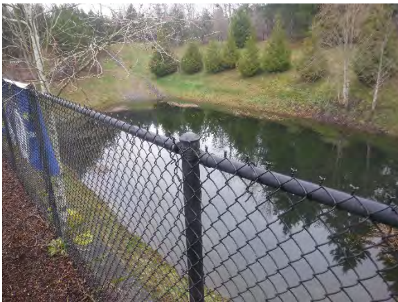
Figure G4.6-7 Drainage pond with restricted access, OMF 151, view east
