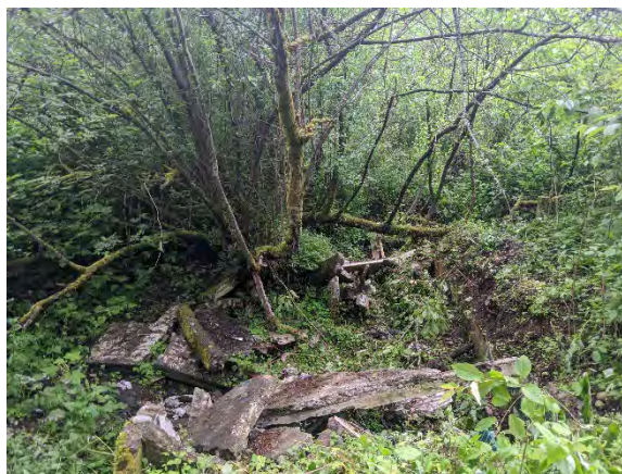
Figure G4.6-29 View of concrete basement with demolition debris, view east
