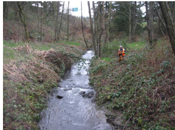
McAleer Creek in the cloverleaf interchange between eastbound SR 104 and northbound I-5, looking upstream from the downstream end of the segment
