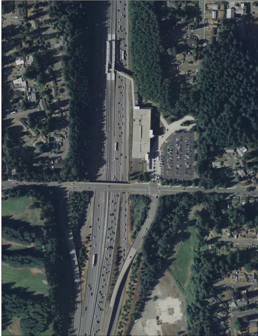
Figure 10. 236th Street SW Interchange
