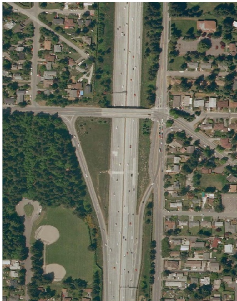
Figure 5. NE 130 th Street Interchange
