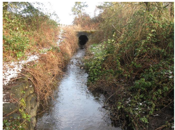
Thornton Creek near 5th Avenue NE, looking upstream toward the outlets of the twin culverts under I-5
