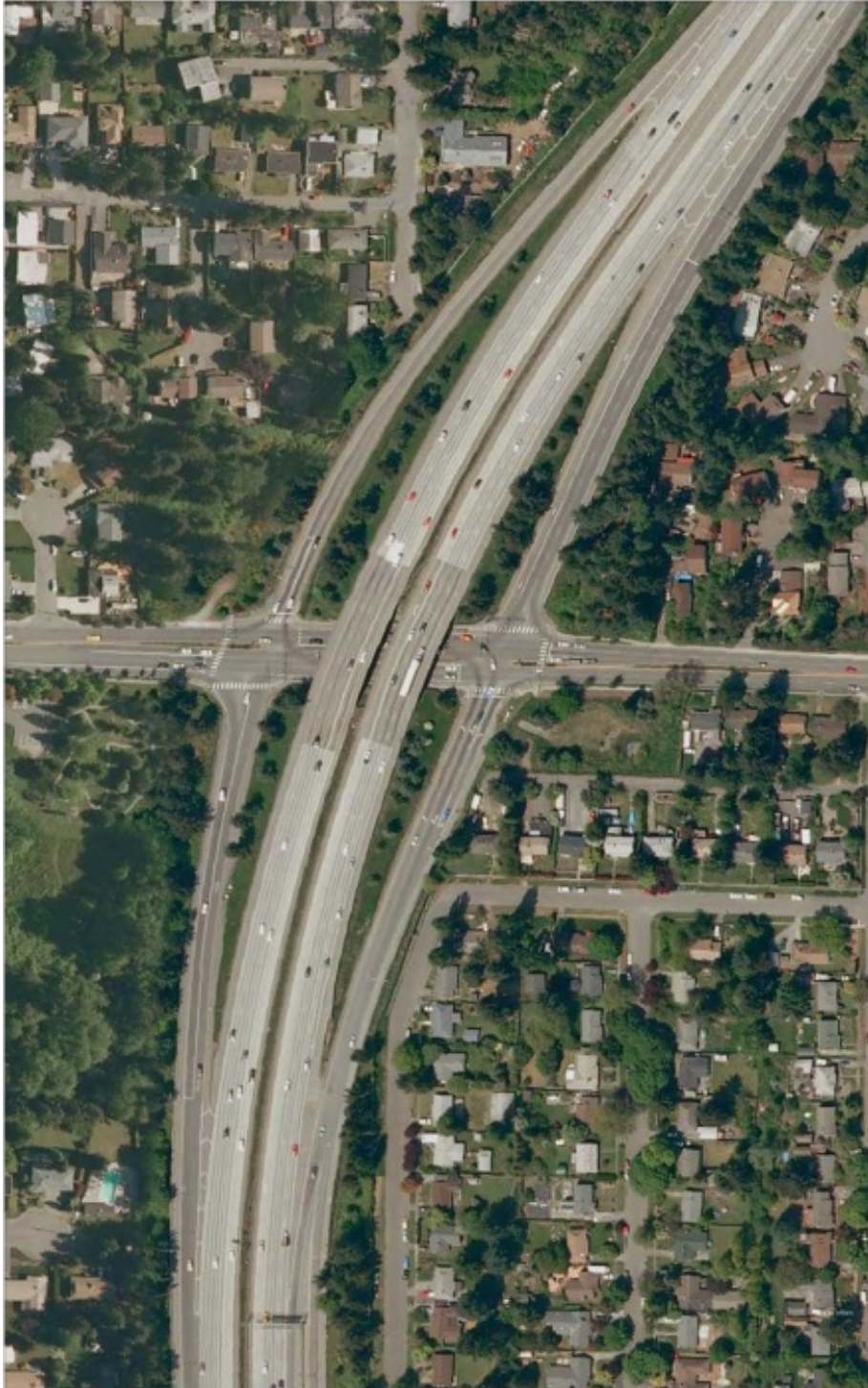
Figure 8. NE 175th Street Interchange
