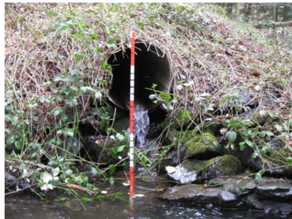
Culvert at confluence of Stream SMT1 with McAleer Creek
