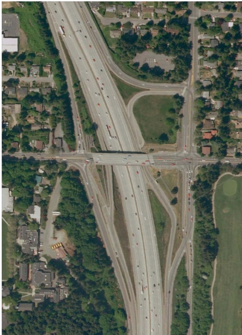
Figure 6. NE 145 th Street Interchange
