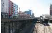
BNSF鐵路軌道上向南看 BNSF railway tracks looking south
