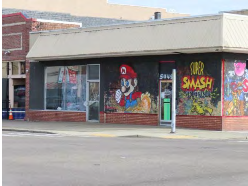
Figure 8.3-1 5447–5449 S Tacoma Way, view northeast
