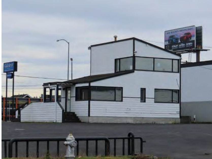
Figure 8.8-3 5802 S Tacoma Way, view southeast
