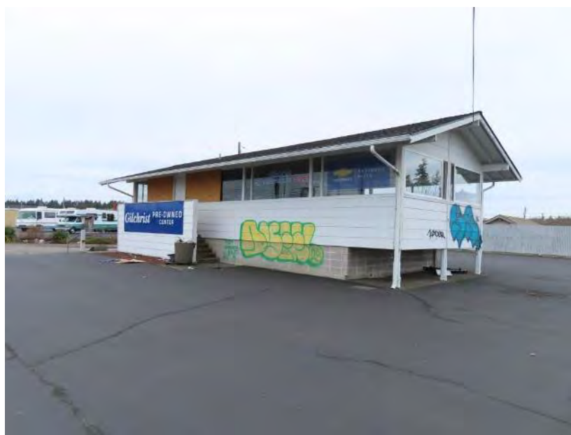
Figure 8.15-1 6001 S Tacoma Way, view northeast
