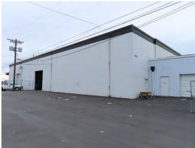
Figure 8.10-2 5802 S Washington Street, view southwest
