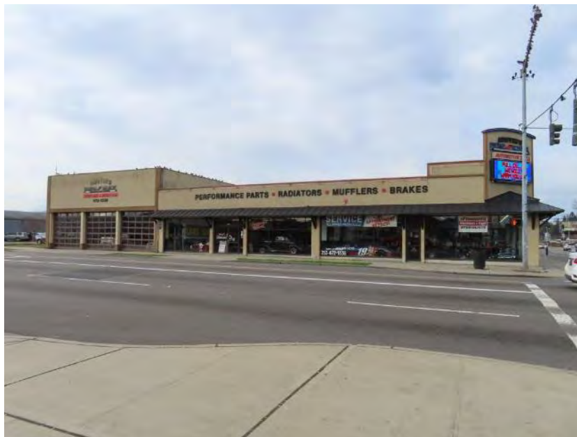
Figure 8.4-2 5602 S Tacoma Way, view west
