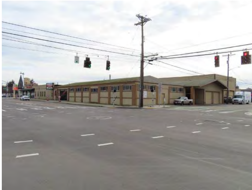
Figure 8.4-3 5602 S Tacoma Way, view southeast
