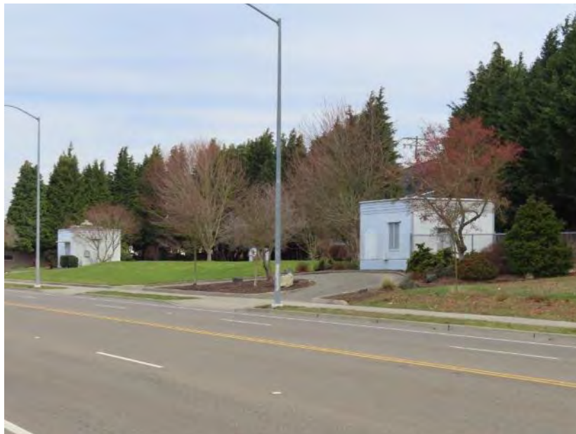
Figure 8.1-1 Wells and wellhouses at 4331 S Tacoma Way, view northeast
