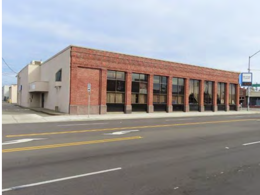
Figure 8.2-2 5448–5450 S Tacoma Way, view northeast
