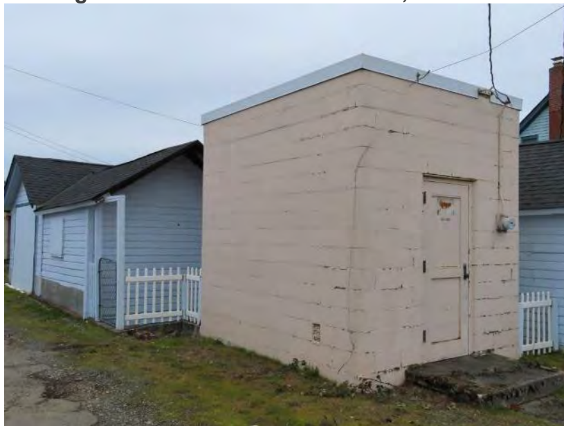
Figure 8.13-2 3509 S 60th Street, view northeast
