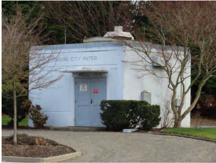
Figure 8.1-2 Wellhouse 11A at 4331 S Tacoma Way, view northeast
