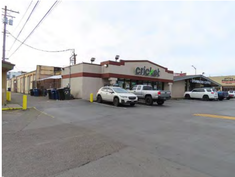
Figure 8.5-1 3512–3514 S 56th Street, view southwest
