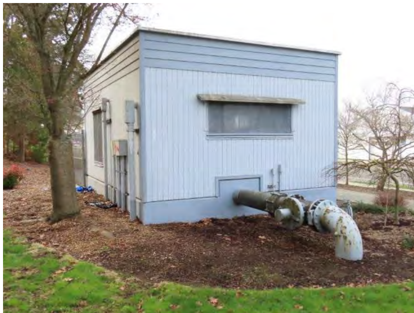
Figure 8.1-3 Wellhouse 6 at 4331 S Tacoma Way, view southwest
