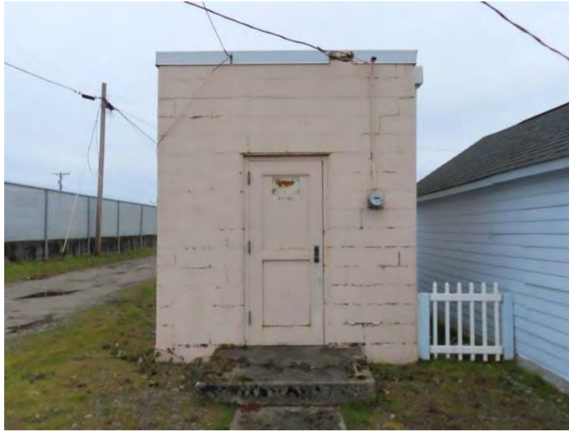
Figure 8.13-1 3509 S 60th Street, view north
