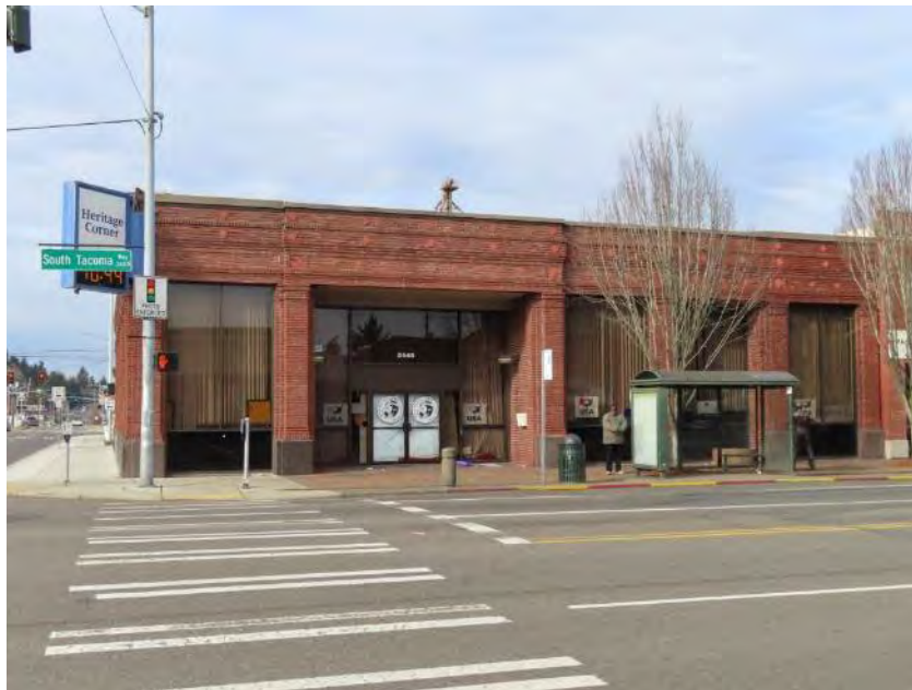
Figure 8.2-3 5448–5450 S Tacoma Way, view west
