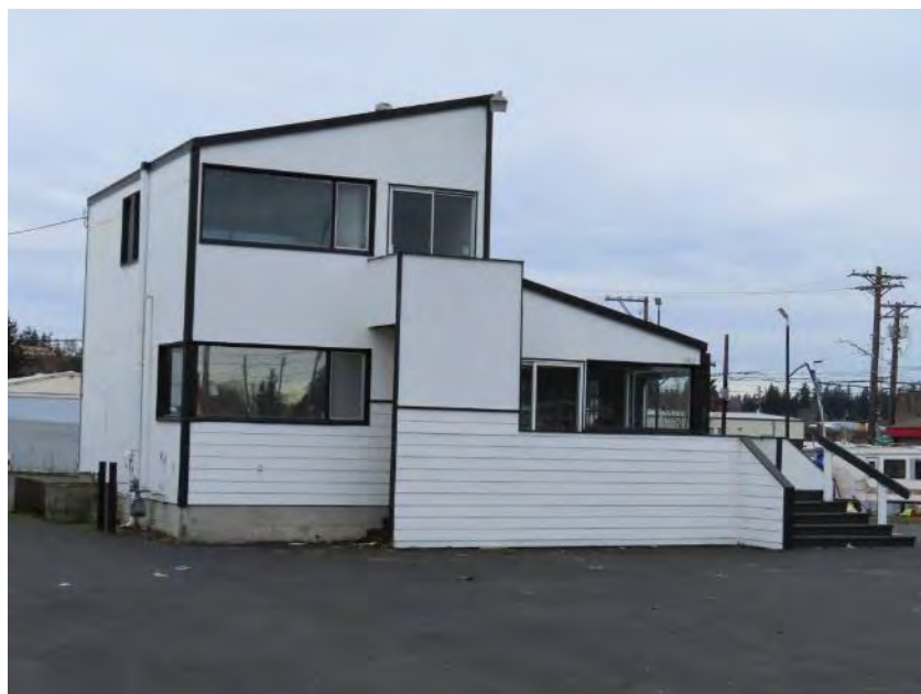
Figure 8.8-1 5802 S Tacoma Way, view west
