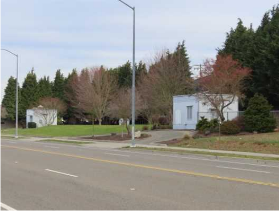
Wells and wellhouses at 4331 S Tacoma Way, view northeast.
