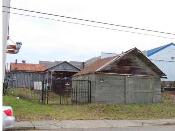
3762 S 60th Street, view east.jpg
