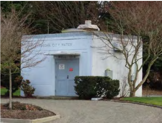
Wellhouse 11A at 4331 S Tacoma Way, view northeast.
