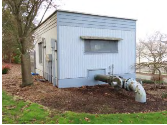
Wellhouse 6 at 4331 S Tacoma Way, view southwest.
