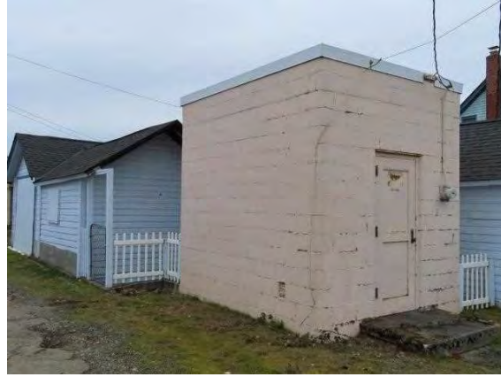
3509 S 60th Street, view northeast.jpg
