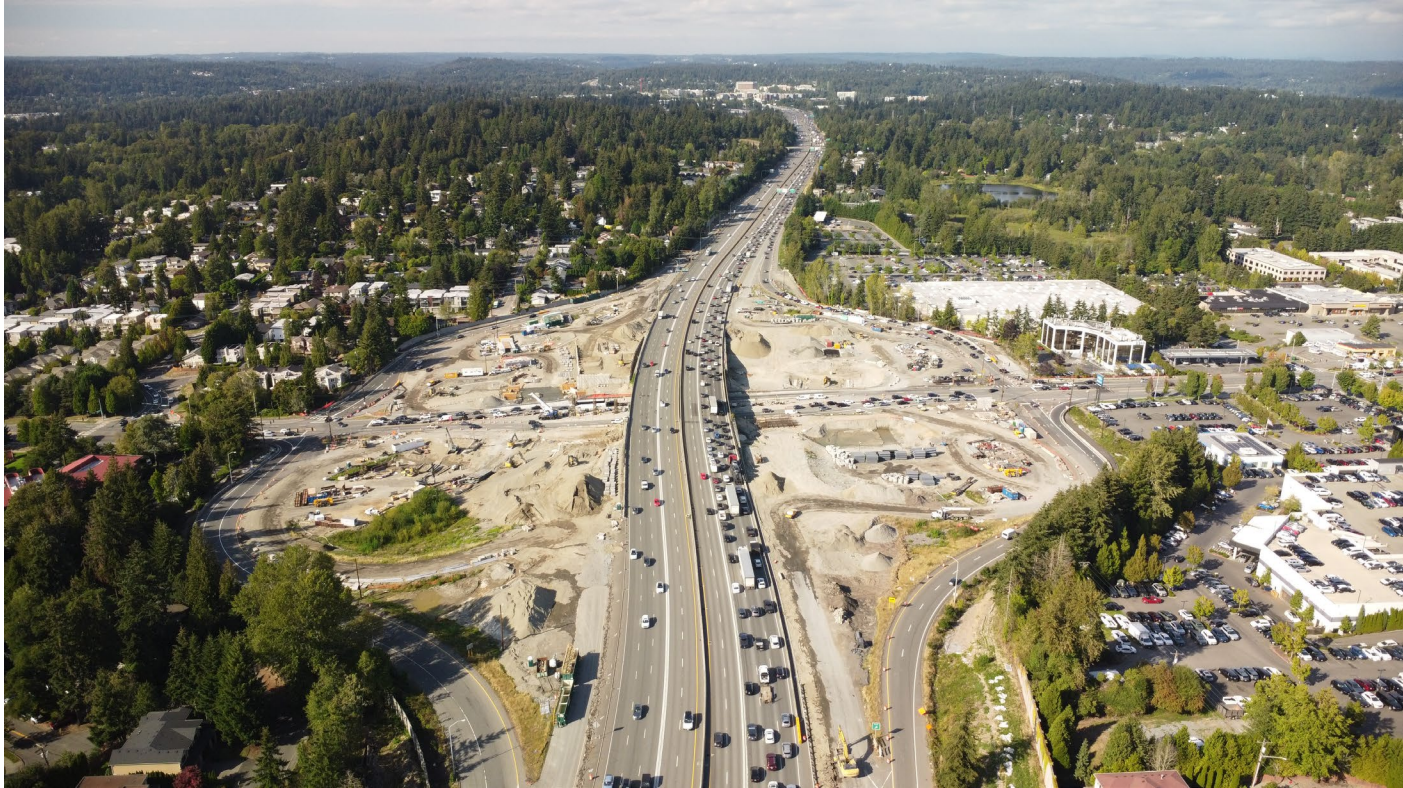
S2: NE 85th Interchange & BRT station looking north (September 2024).
