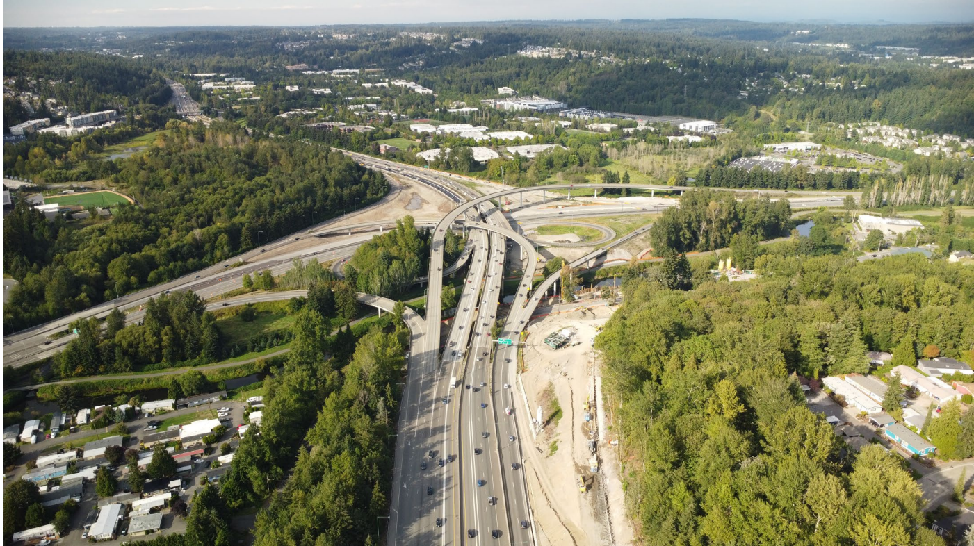
S2: SR 522/I-405 Interchange & BRT station looking north (September 2024).
