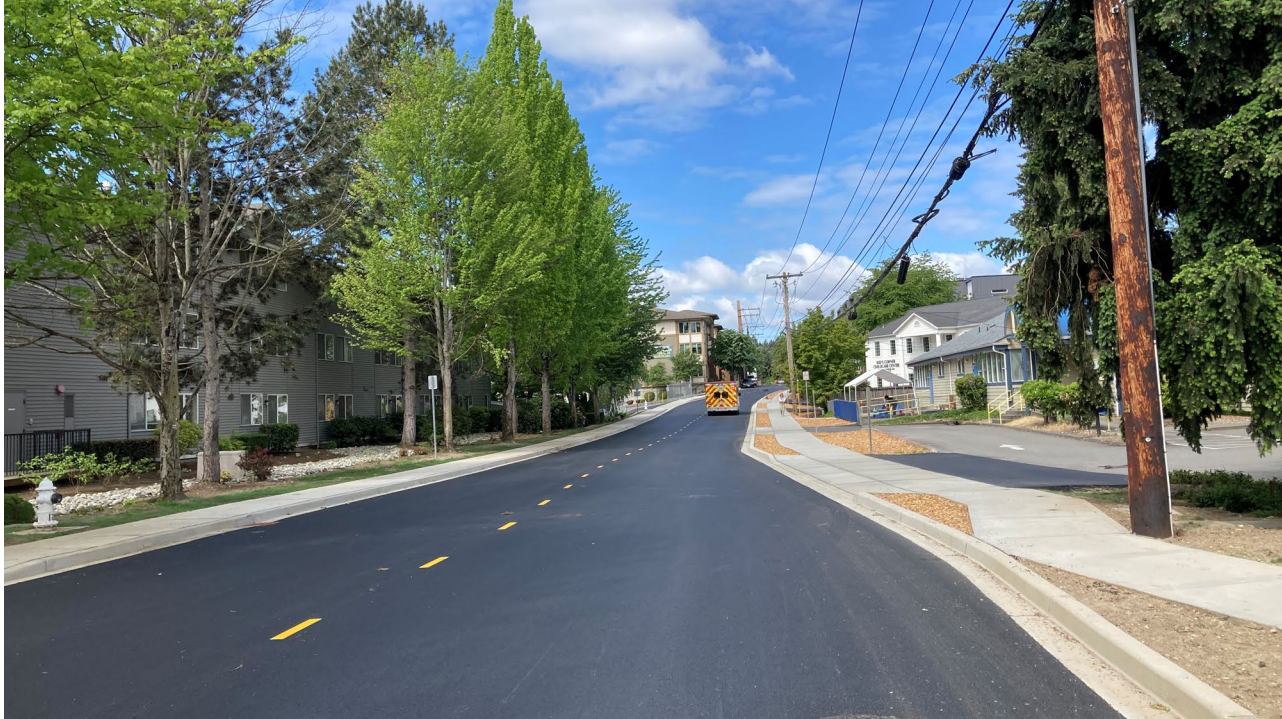
S3: NE 185 th St reconstruction looking west (May 2024)
