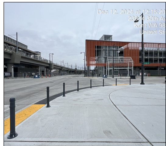
Bollards Installation at 236th St. Des Moines
