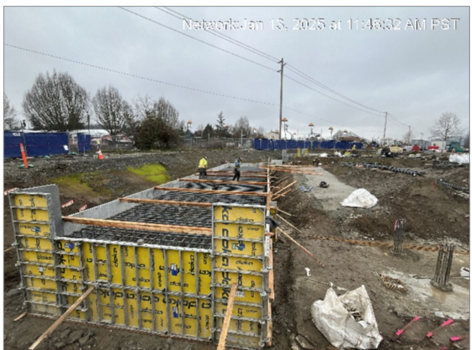
Forming & pacing pile caps/grade beams at Sumner
