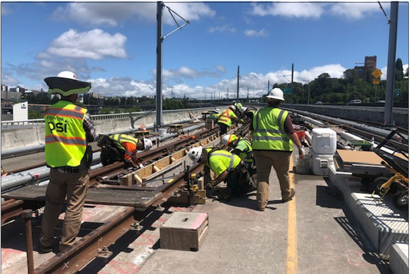
Track construction on previous I-90 HOV Lanes
