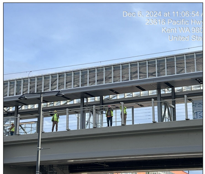
Egress Extension Install at Kent Des Moines Station
