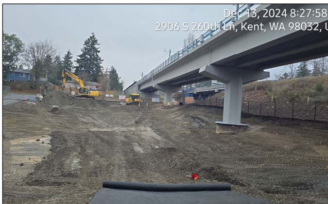
Structure C- Pond E Excavation and Grading
