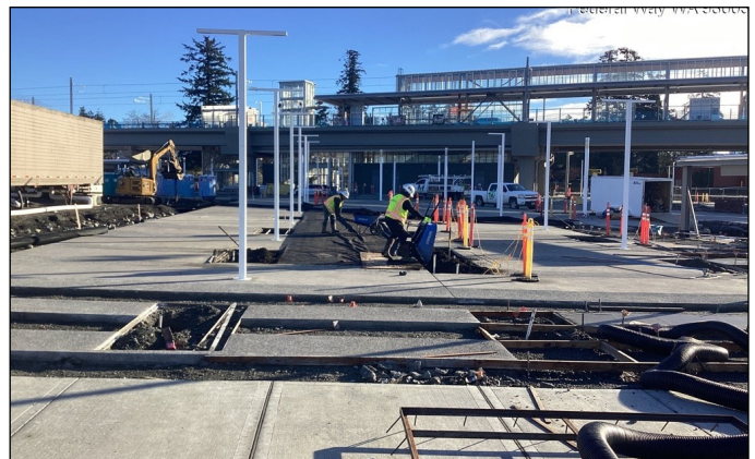
Federal Way Downtown-Tree Pit Topsoil
