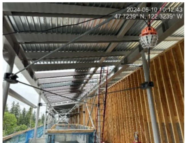
Platform roofing installation
