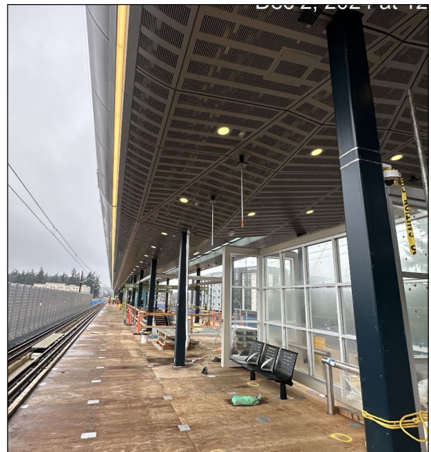
Plaza Slab Construction at Downtown Redmond Station
