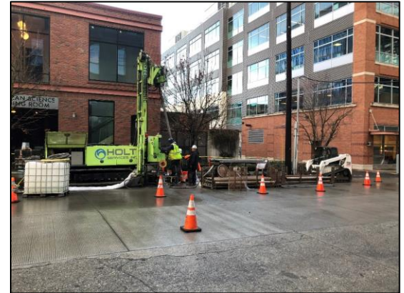
Geotechnical drilling rig in South Lake Union.
