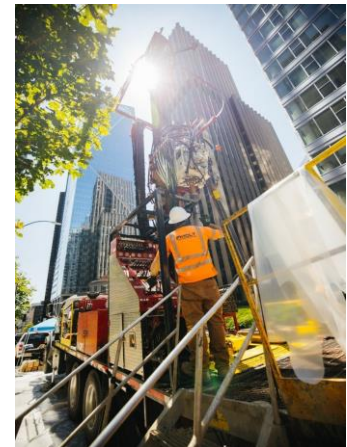
Geotechnical drilling rig in Downtown Seattle.
