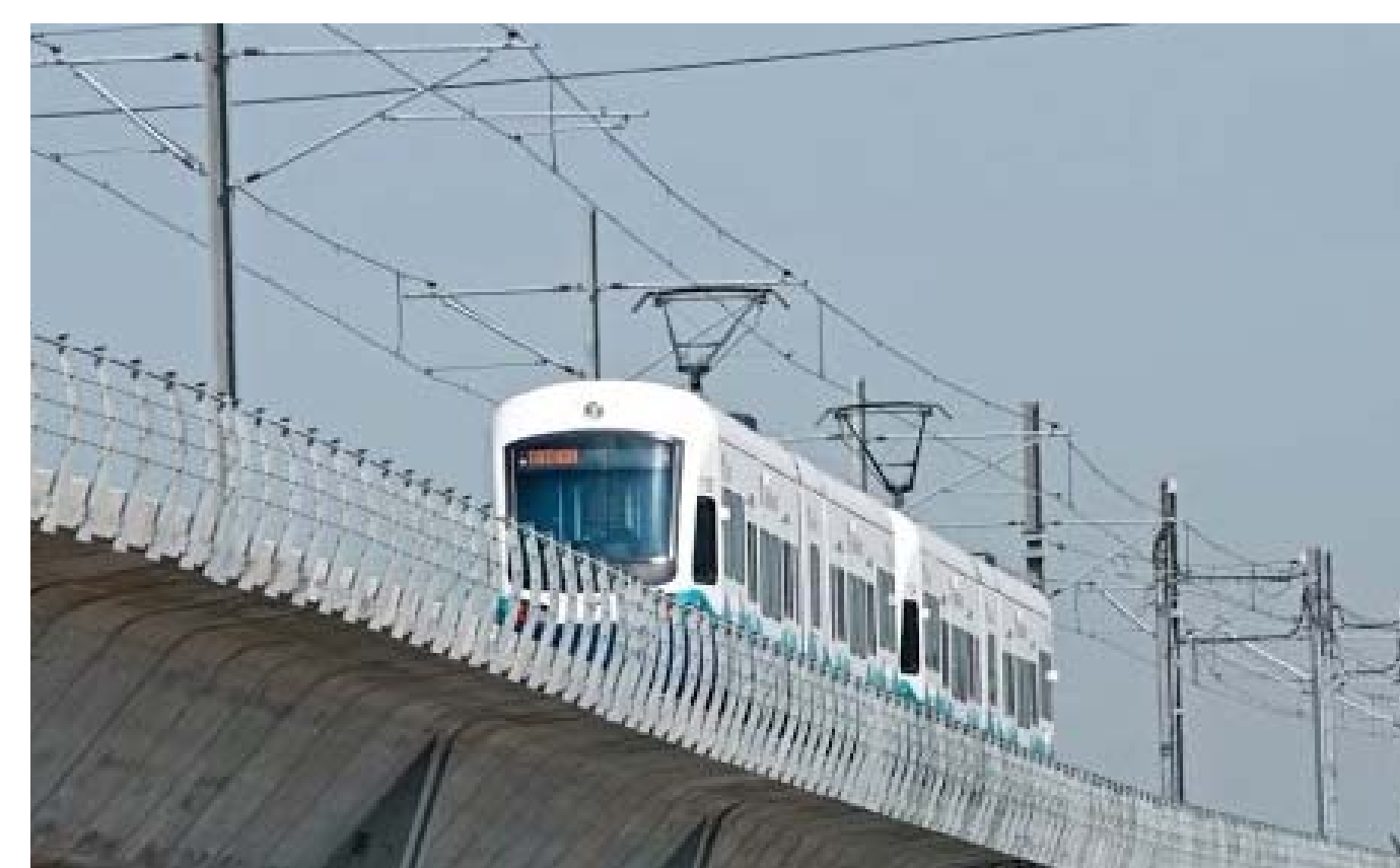
16. POWER & COMMUNICATION POLES
