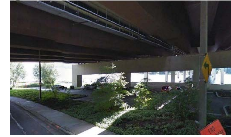
Enatai Beach Park – Seismic improvements and project staging
