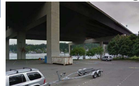
Mercer Island Boat Launch – Seismic improvements
