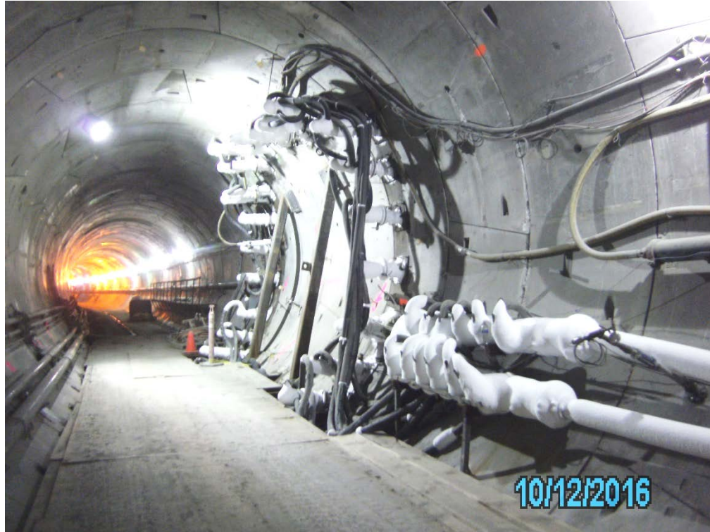
Soil freezing technology to stabilize soil
