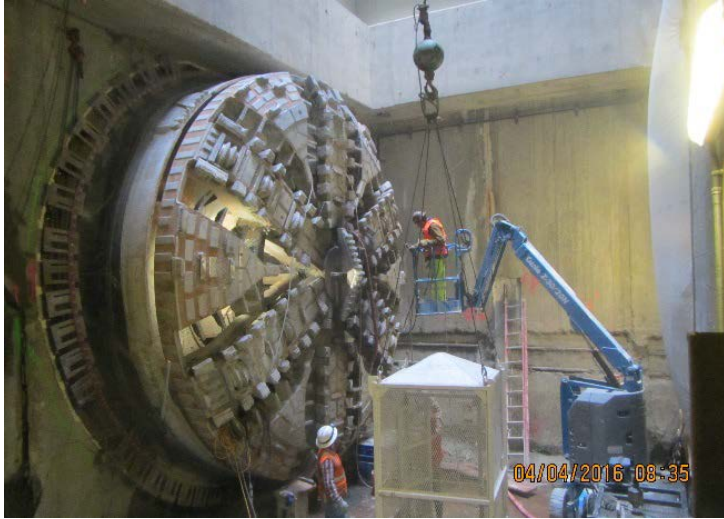
Tunnel Boring Machine (TBM)
