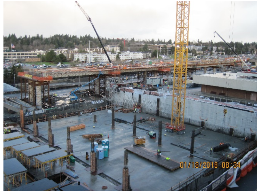
450 stall parking garage; elevated guideway in background
