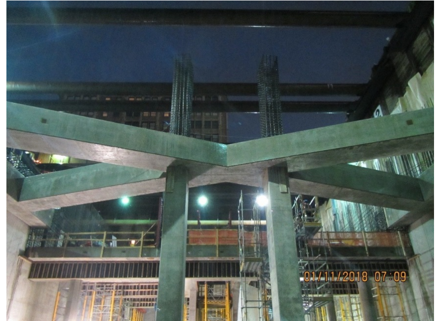
Internal bracing for station walls
