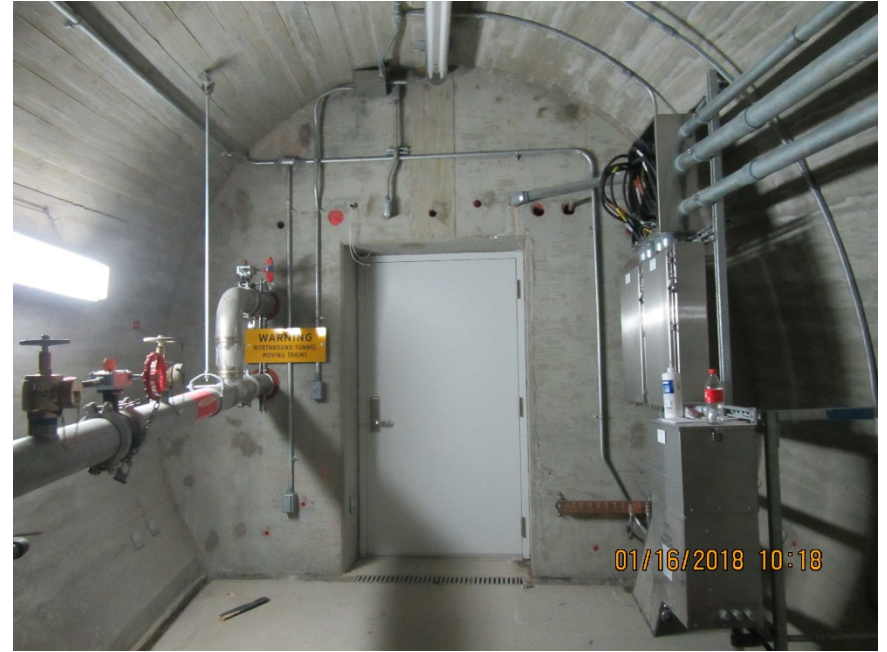
Finished cross passage
