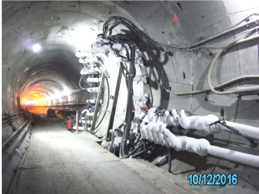
Ground Freezing to Stabilize Soils
