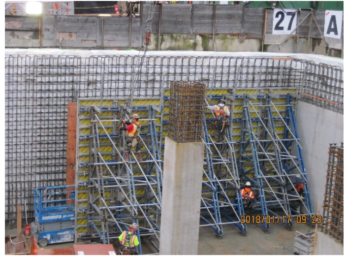
Formwork for station walls
