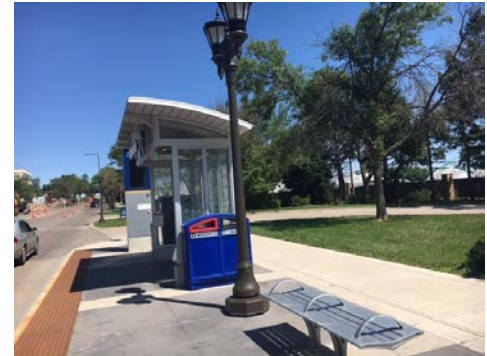
Example BRT – Minneapolis Metro A Line
