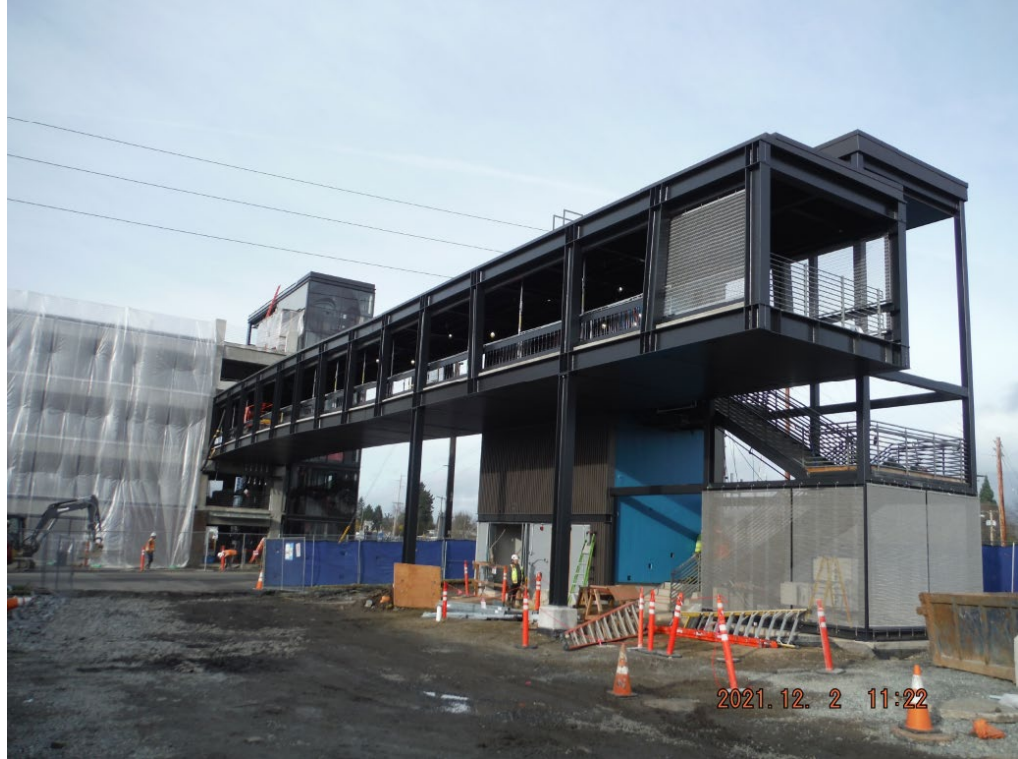
Bridge screening installation - December 2nd
