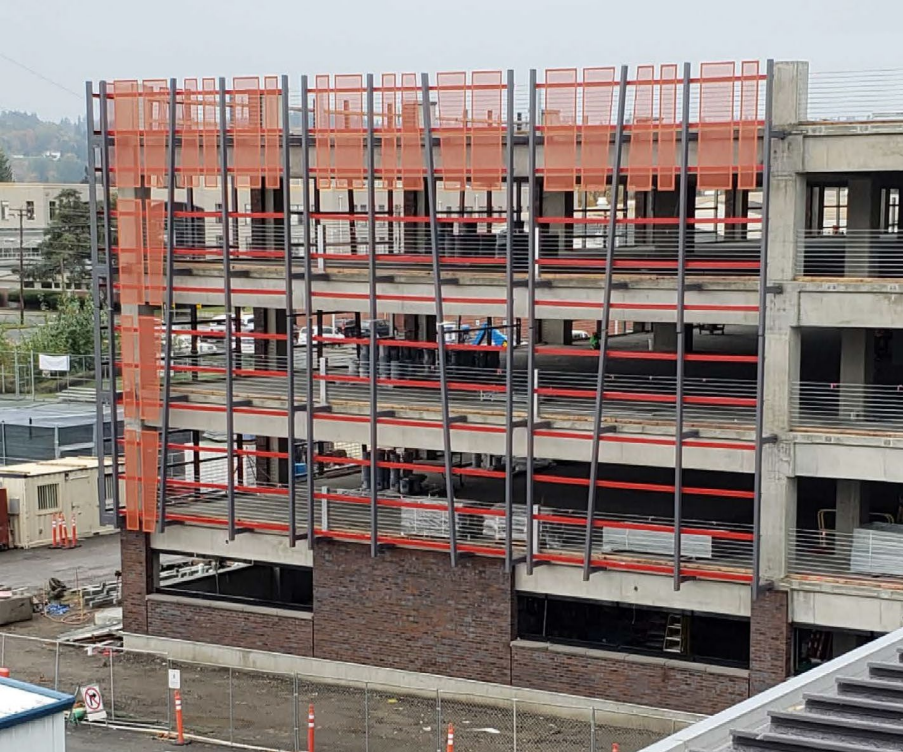
Garage facade panel installation
