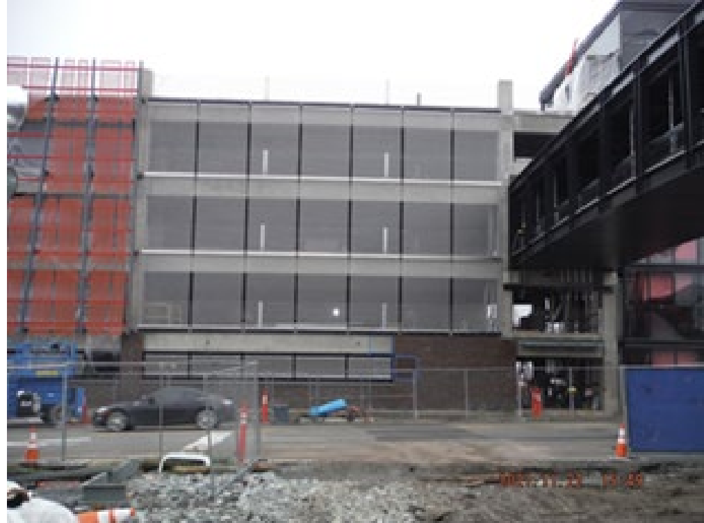
Garage facade screening.
