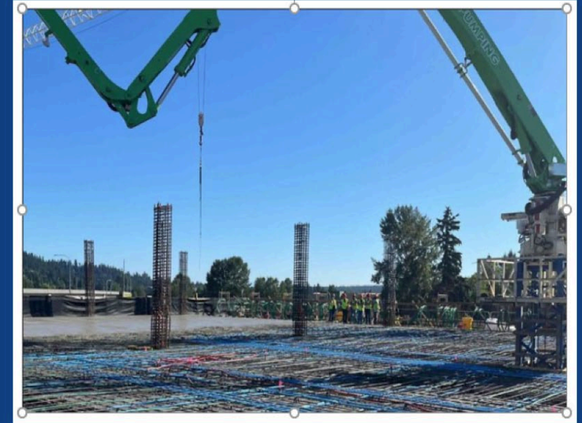
Downtown Redmond Link Extension Garage Construction
