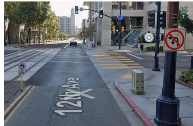
Figure: Example of eye-level “NO LEFT TURN” signage and delineator
